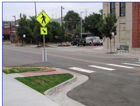
Constructing Curb Bump Outs
