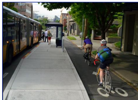
Floating Bus Stop Construction
