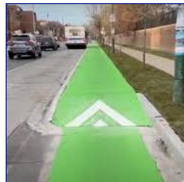
Raising Bike Lanes to Sidewalk Level
