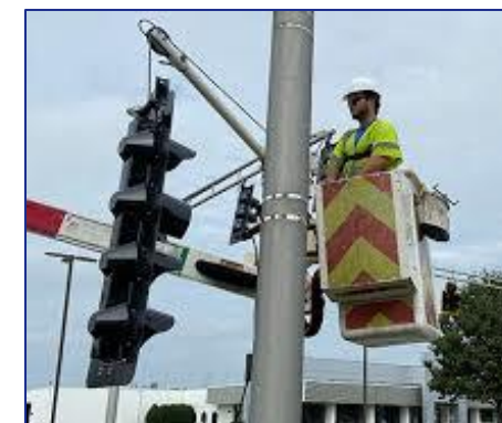
Install New Traffic Signal
