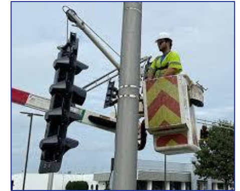
Install New Traffic Signal
