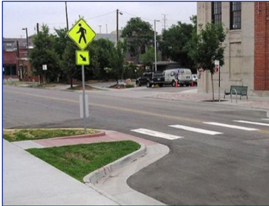
Constructing Curb Bump Outs
