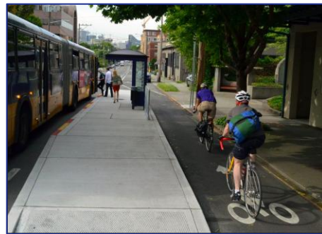
Floating Bus Stop Construction
