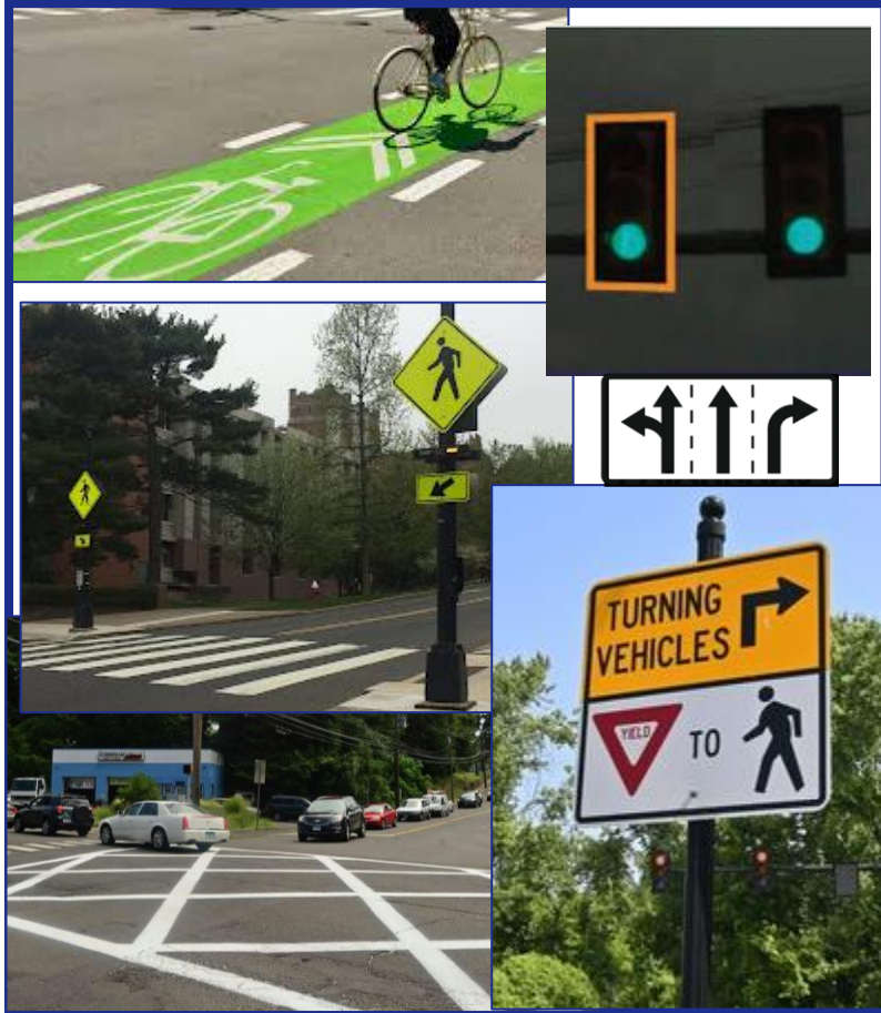
Visibility, Awareness, and Compliance Improvements
