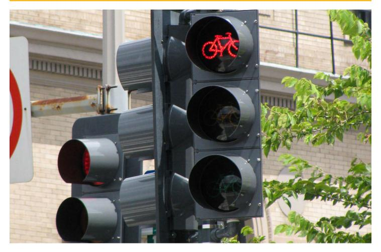
Bicycle signals and beacons facilitate bicyclist crossings of roadways. Bicycle signals make crossing inersections safer for bicyclists by clarifying when to enter an intersection and by restricting conflicting vehicle movements.
