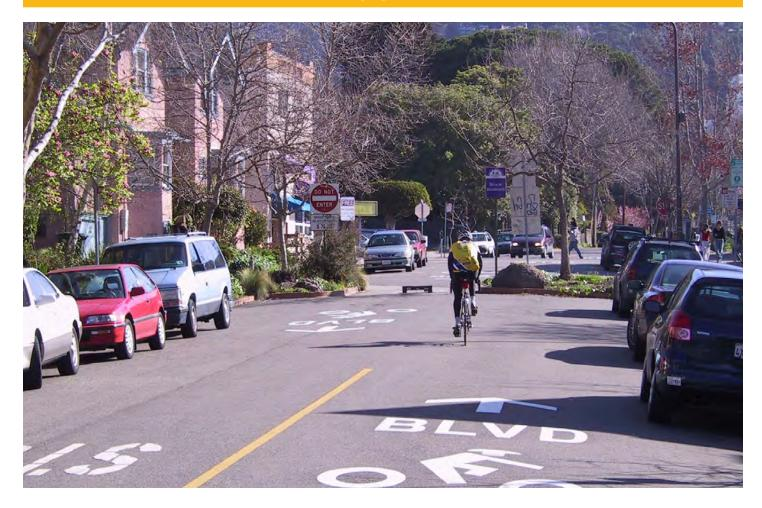
Bike boulevards are streets with low motorized traffic volumes and speeds, designated and designed to give bicycle travel priority. Bike boulevards use signs, pavement markings, and speed and volume management measures to discourage through trips by motor vehicles and create safe, convenient bicycle crossings of busy arterial streets.
