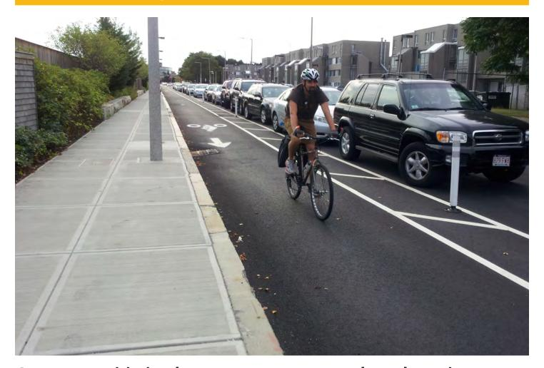
Separated bike lanes are at street level and use a variety of methods for physical protection from passing traffic. A separated bike lane may use a parking lane or other barrier between the bike lane and the motor vehicle travel lane. Benefits include a reduced risk of "dooring," preventing double-parking, reducing risks from motorists entering/exiting parking spaces, and being more comfortable for bicyclists of all levels and ages.
