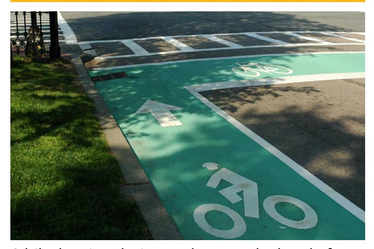
A bike box is a designated area at the head of a traffic lane at a signalized intersection that provides bicylists with a safe and visible way to get ahead of queuing traffic during the red signal phase. They increase visibility of bicyclists and reduce signal delay for bicyclists. Bike boxes that extend across an entire intersection can also facilitate bicyclist left turn positioning during red lights.
