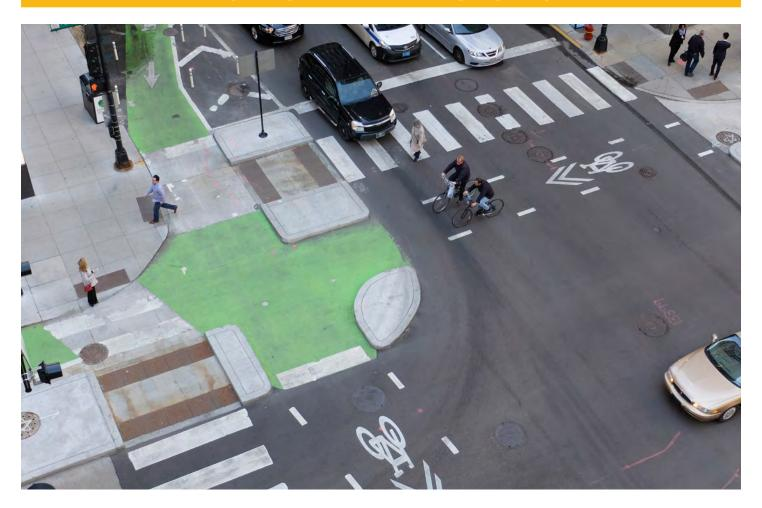
Protected intersections are extensions of existing curblines that provide bicyclists with vertical and horizontal separation from motor vehicles through an intersection. They are typically constructed of concrete, however may also use quick-build materials as interim facilities.
