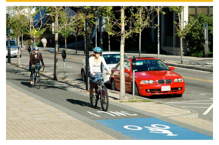
Raised separated bike lanes are bicycle facilities that are vertically separated from motor vehicle traffic. Many are paired with a furnishing zone between the bike lane and motor vehicle travel lane and/or pedestrian area. Benefits include that motorists are kept from easily entering and it is more attractive to a wider range of bicyclists at all levels and ages than less separated facilities.
