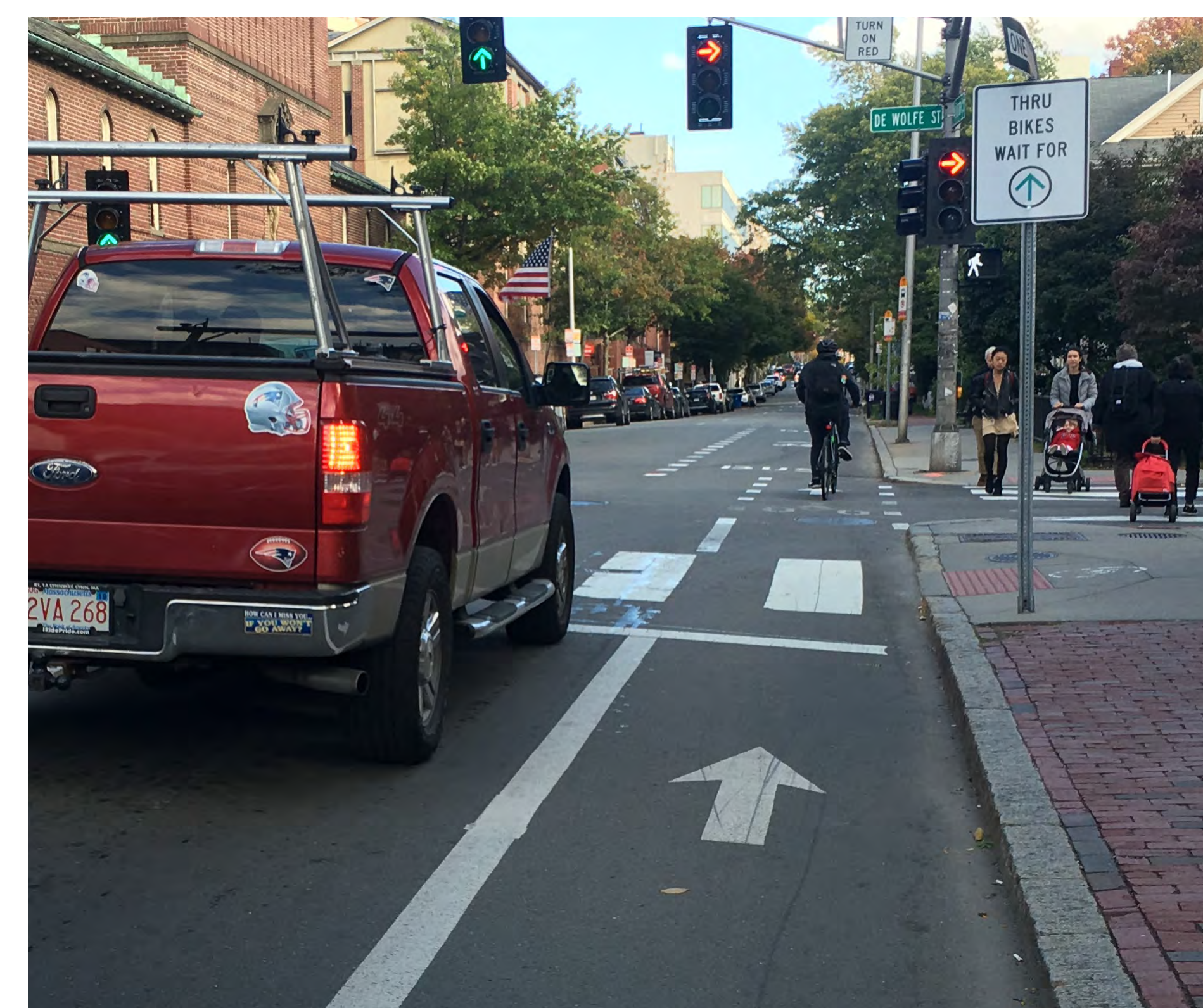
Mt Auburn St bike lane widening, bike signal
