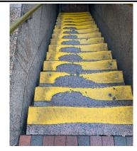
Worn out tactile tread warning surface cover on staircase
