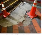
Cracked floor tile & damaged patch work
