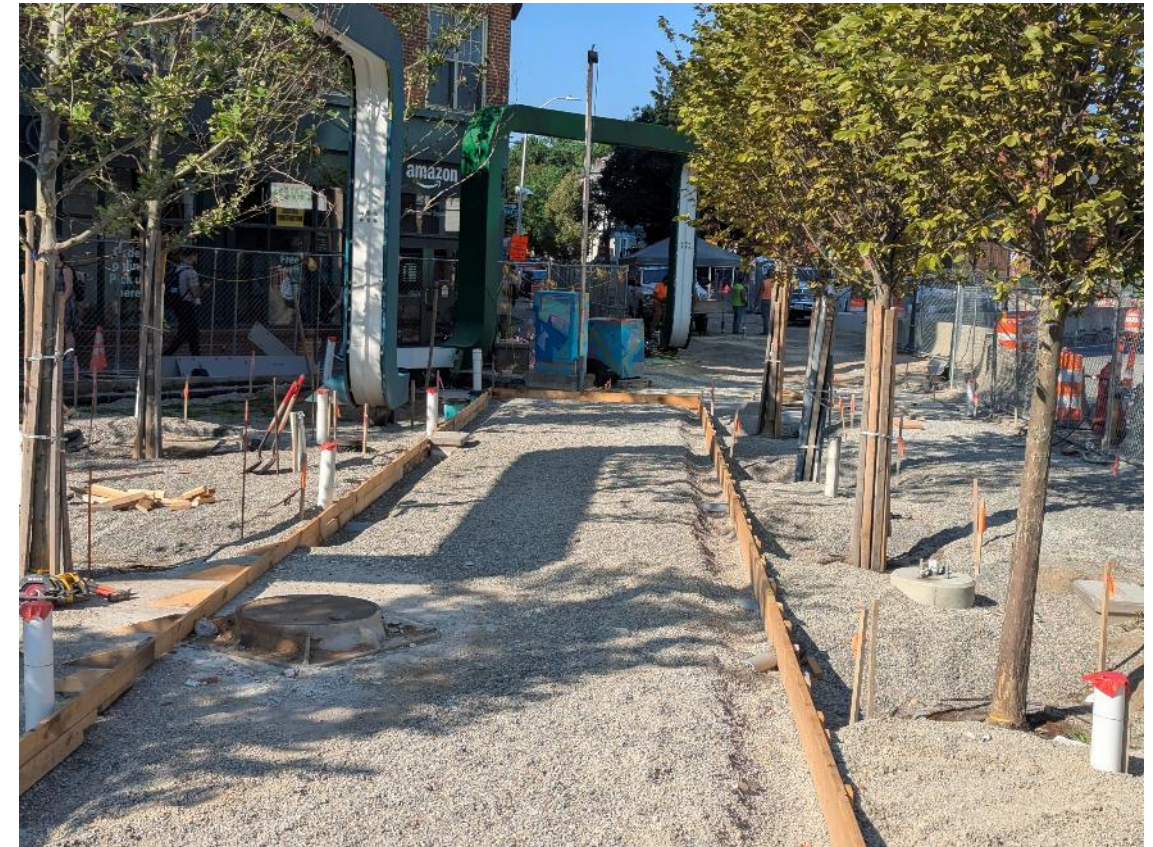
Image: Plywood forms set in Carl Barron Plaza. Forms align with future pathways around plaza toward bus terminal.
