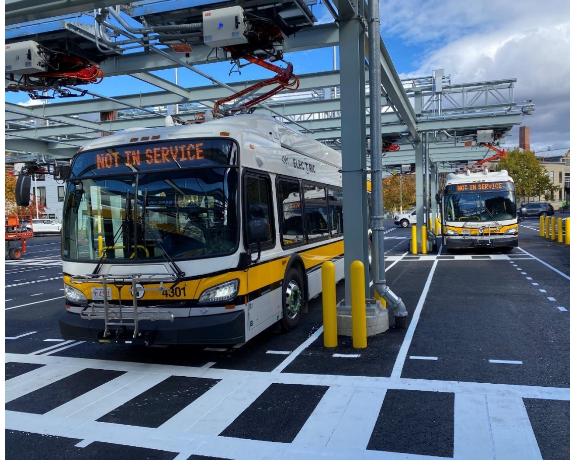
New Battery Electric Outdoor Charging Facility
