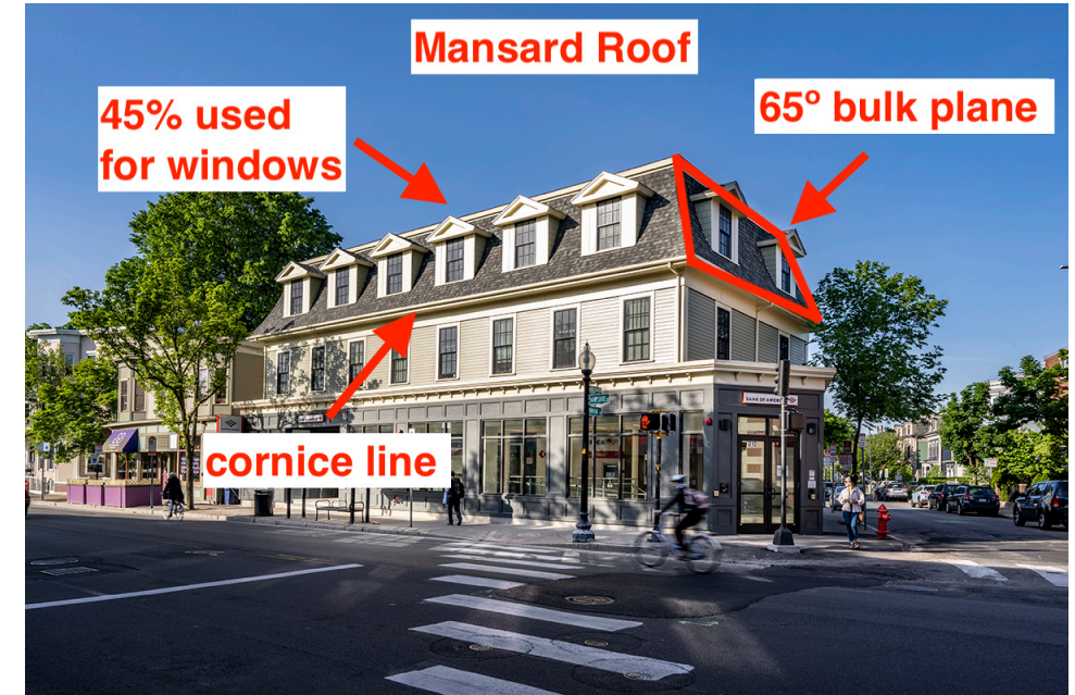
212 Hampshire Street Mansard Roof
