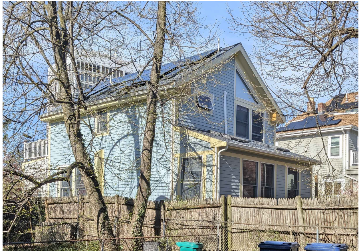
6. REAR AND SIDE VIEWS OF EXISTING BUILDING TO BE DEMOLISHED
