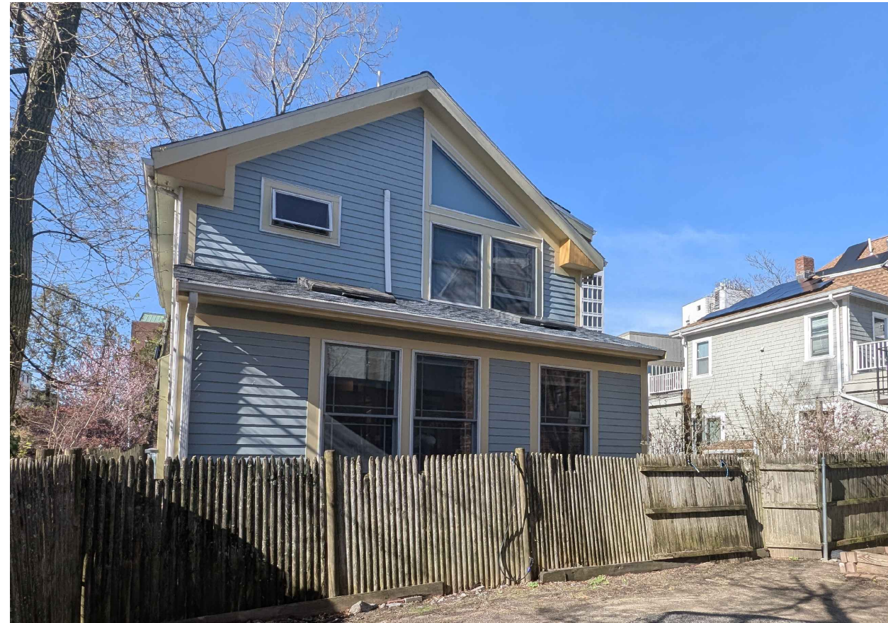
5. SIDE VIEW OF EXISTING BUILDING TO BE DEMOLISHED
