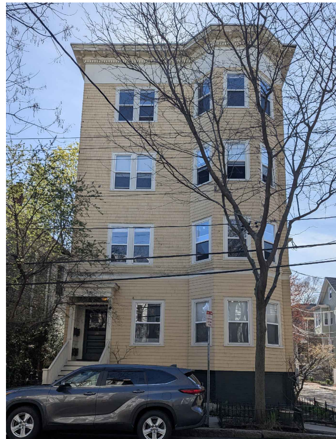
NEIGHBORING BUILDING AT 28 ESSEX ST.
