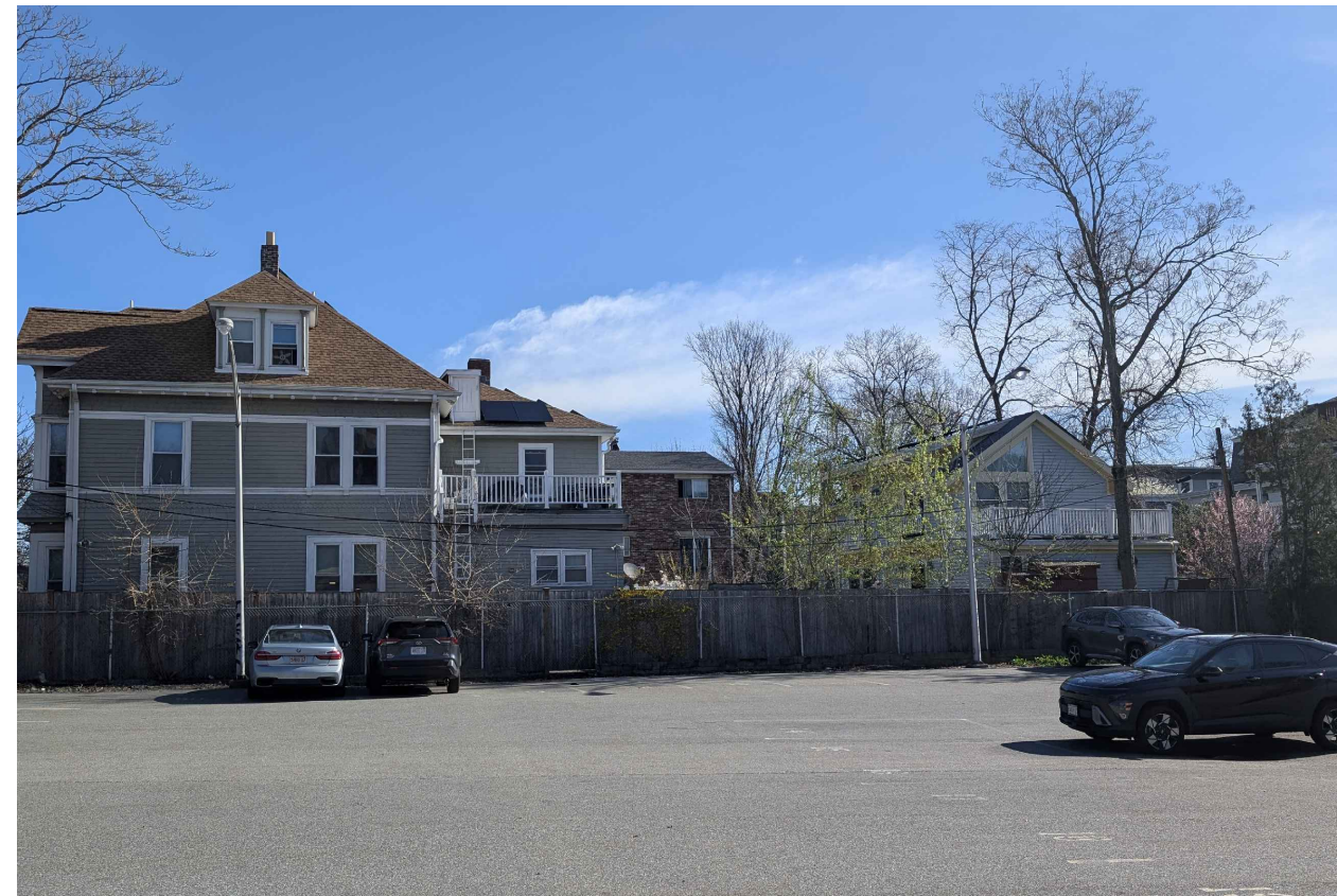
1. SIDE VIEW OF EXISTING BUILDING TO REMAIN
