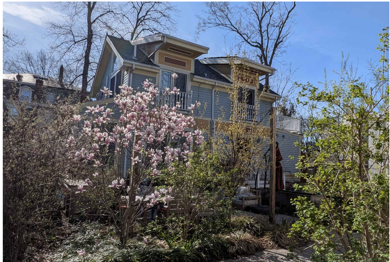
4. FRONT VIEW OF EXISTING BUILDING TO BE DEMOLISHED
