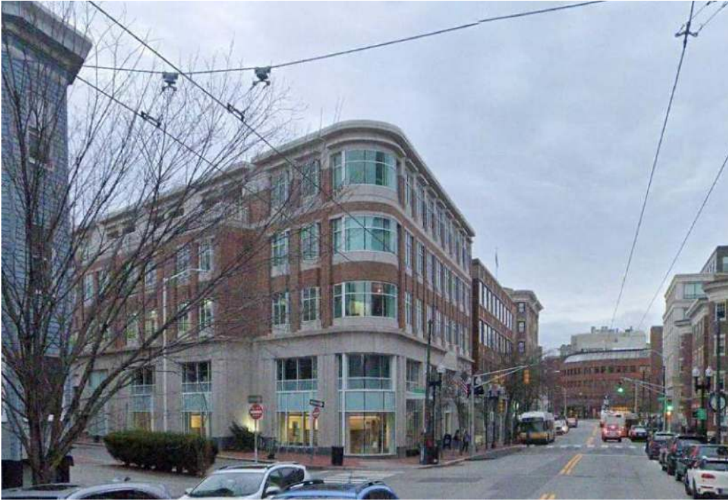
5. View from the edge of the reduced APE along Mt Auburn Street facing east-southeast towards the host structure.
