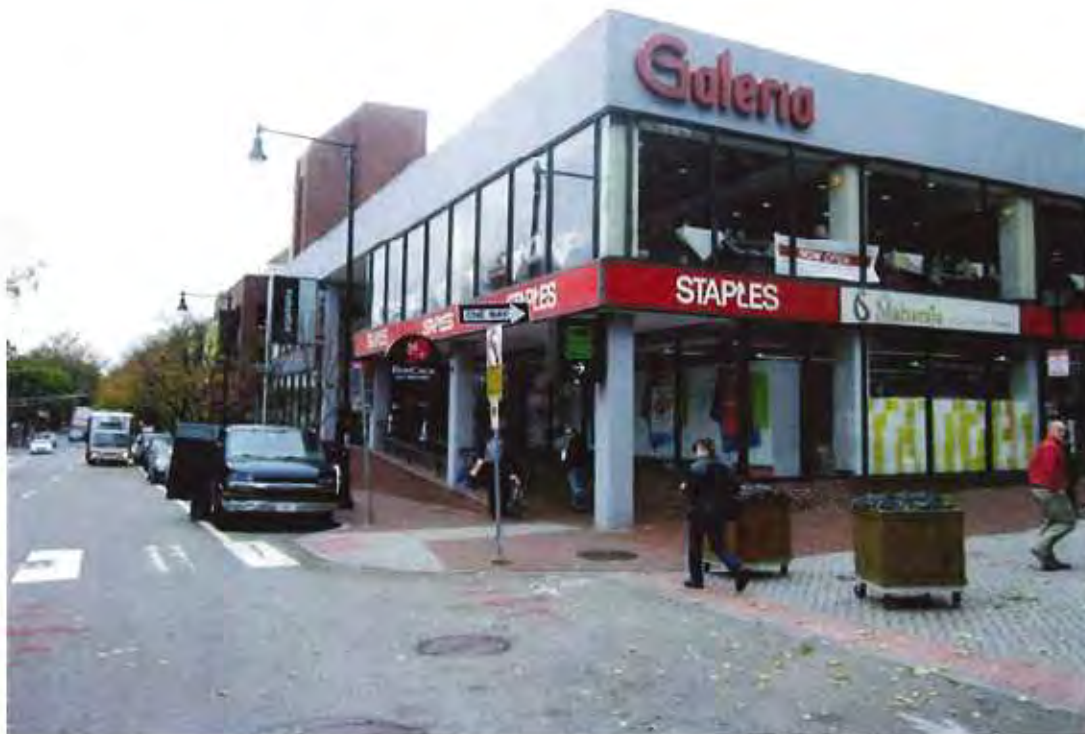
Fig 2 – View of N.E. corner of building
