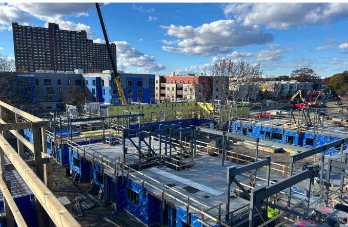
Jefferson Park Federal, North Cambridge, 278 units — Status: under construction.
