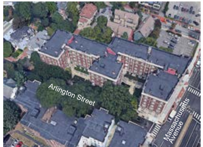
At its corner facing the intersection of Massachusetts Avenue and Arlington Street, this mixed-use building has a zero setback and ground floor retail uses. Its wings facing Arlington Street are set back to relate to the street's typical residential setbacks. Entry forecourts between the wings open onto the tree-lined street, connecting semi-public space within the site to the public realm.
