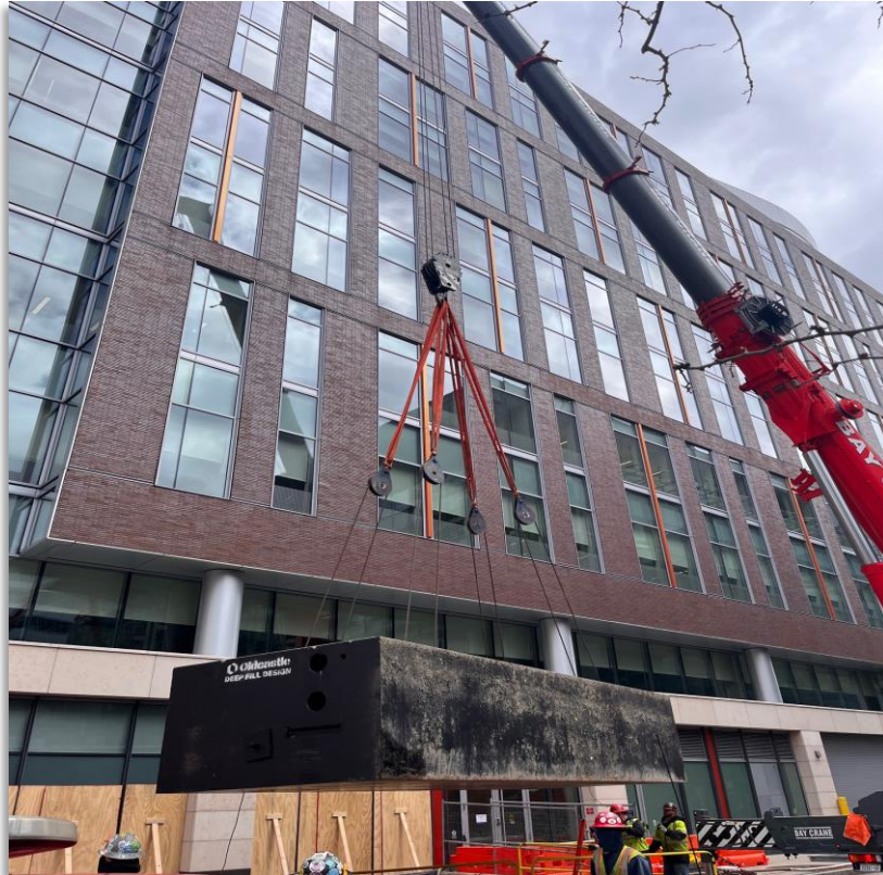
Vault installation using a crane to lower the vault into place
