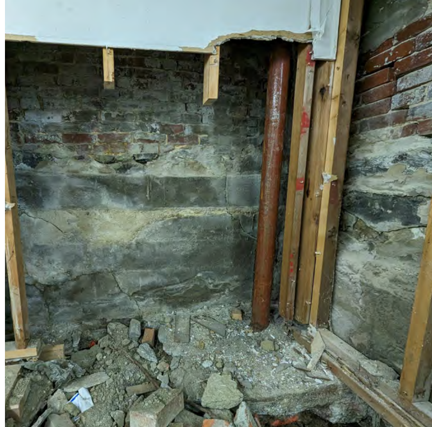
PREVIOUS UNDERPINNING/ REPAIR AT SE CORNER
