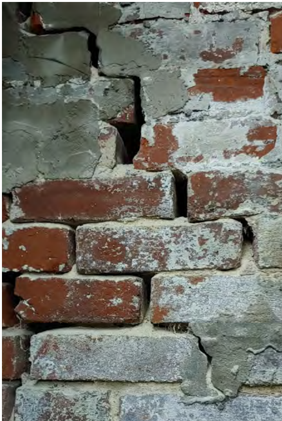
DETERIORATED MASONRY AT FOUNDATION WALL
