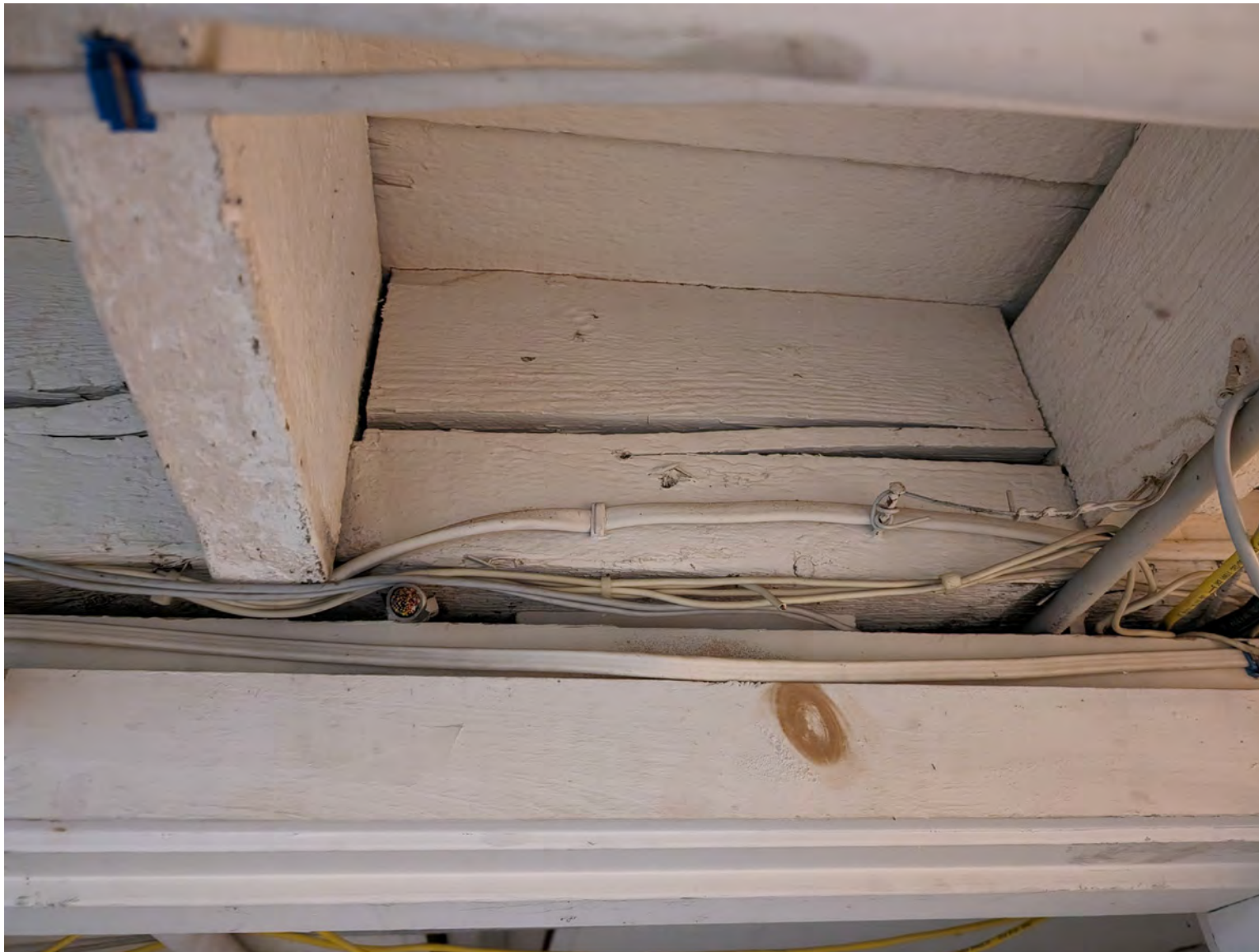
COMPROMISED FLOOR FRAMING BEAM
