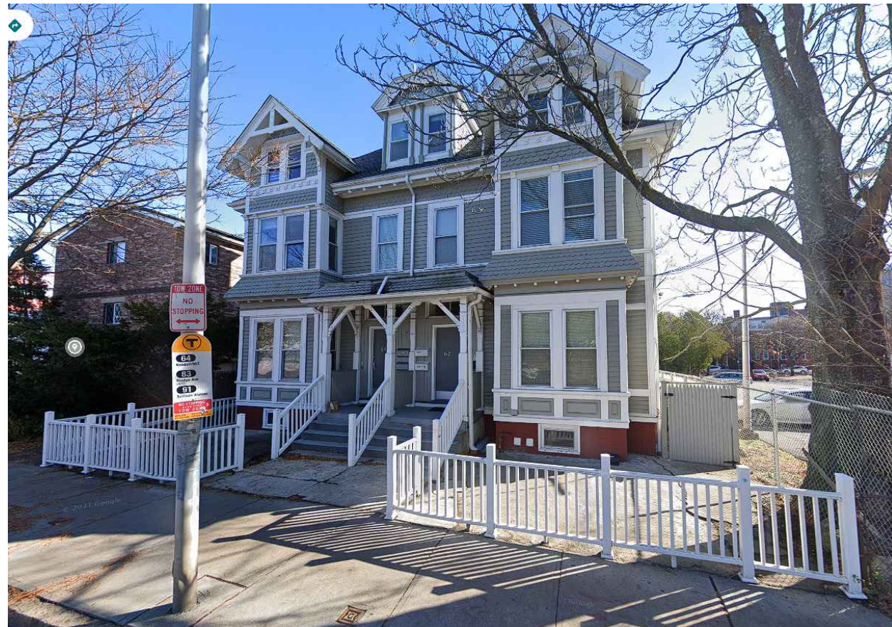
2. FRONT VIEW OF EXISTING BUILDING TO REMAIN
