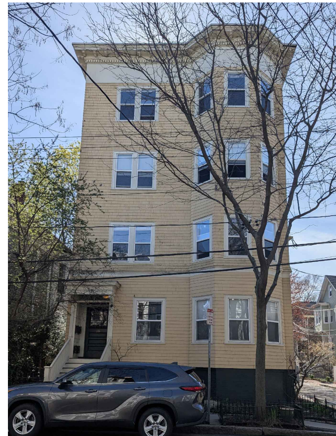
NEIGHBORING BUILDING AT 28 ESSEX ST.
