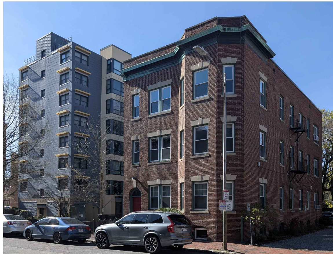
NEIGHBORING BUILDING 55 ESSEX ST (JFK APARTMENTS) & 252 HARVARD ST
