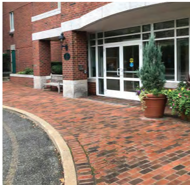
Concrete curb with brick paving at building entrances
