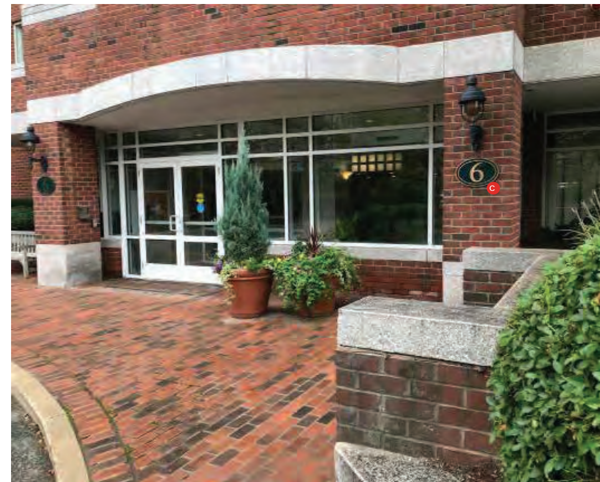
C Building address at entry door
