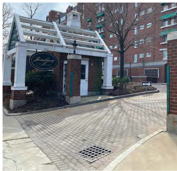
Granite curb with concrete pavers at entrance drive
