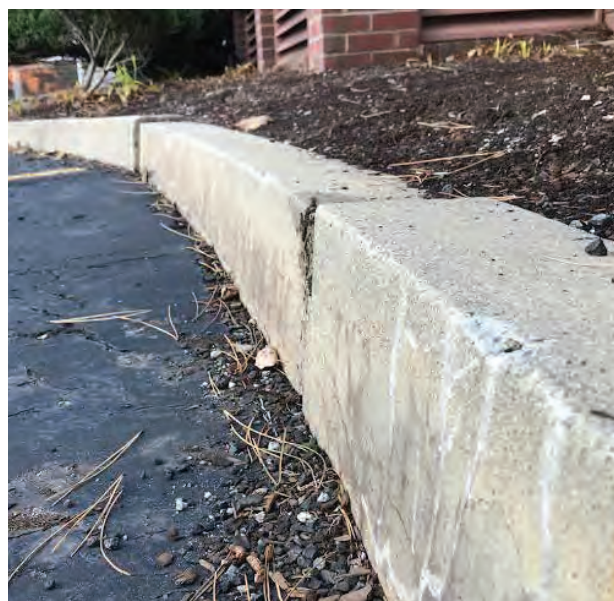
Concrete curb with asphalt paving at parking areas
