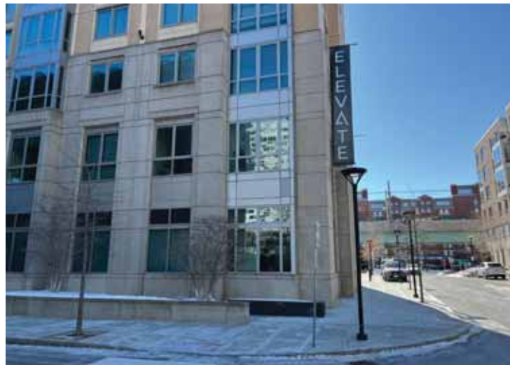
D.2 Corner of Glassworks and Leighton Street
