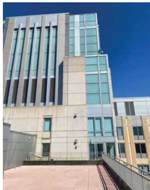
D.8 Existing Level 21 Terrace
