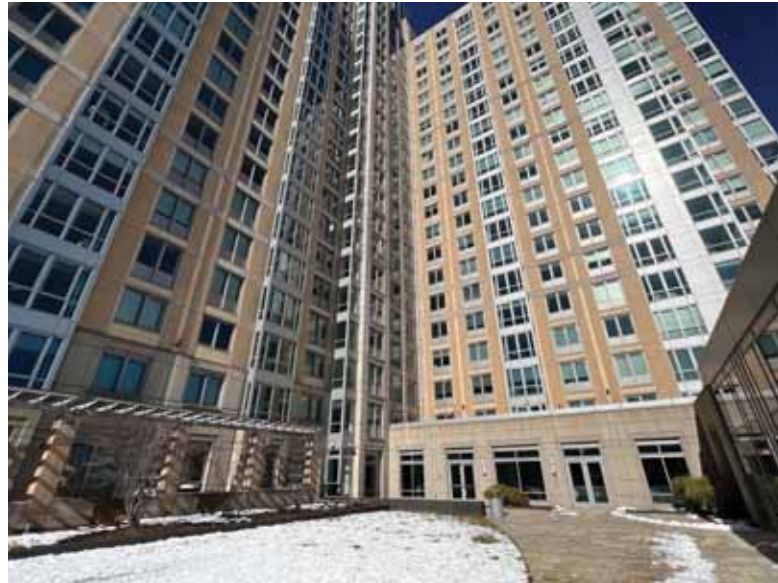
D.4 Existing Courtyard Looking Northwest
