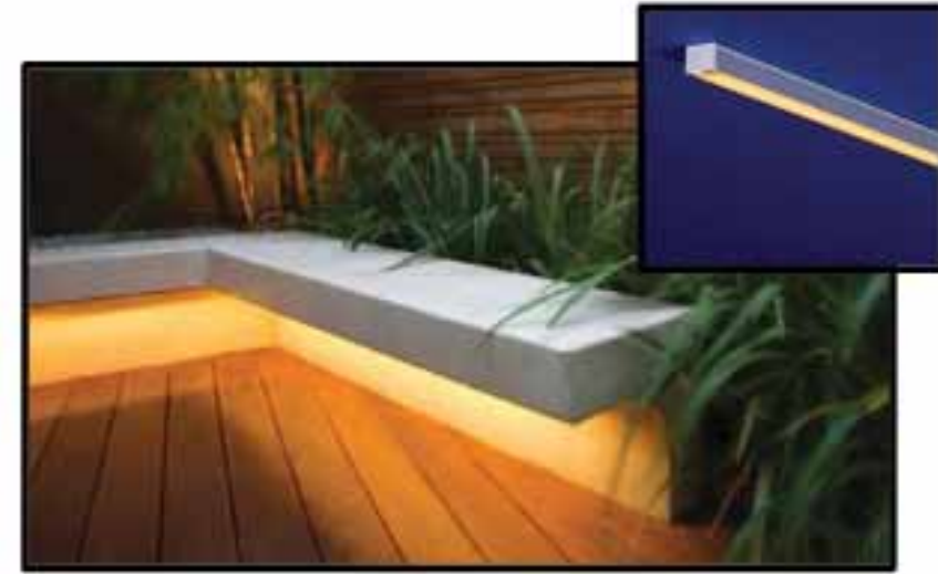
Dimmable, programmable color-changing LED lighting to be integrated under benches and controlled automatically via astronomic time clock
