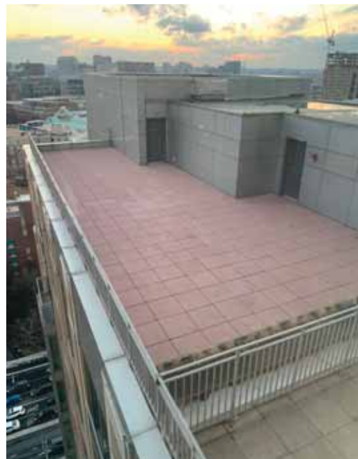
D.7 Existing Level 21 Terrace
