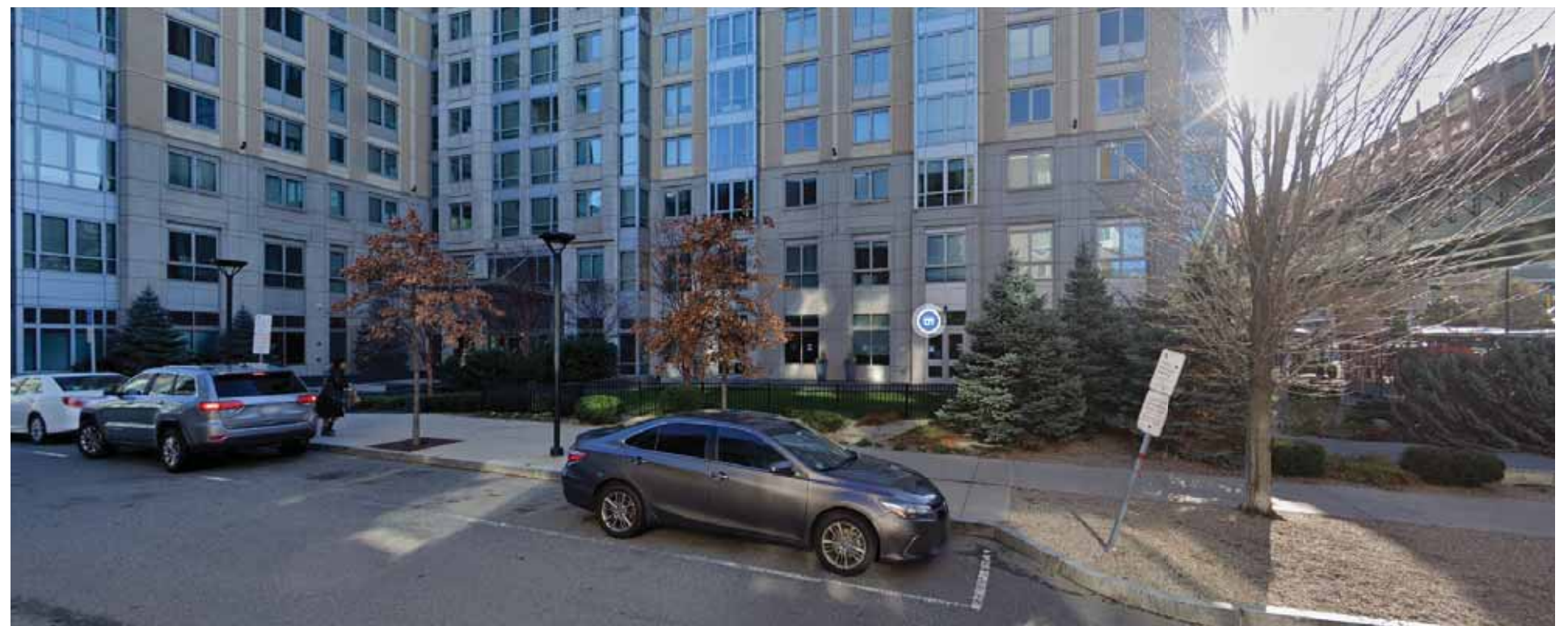
U.2 VIEW FROM LEIGHTON STREET OF WEST FACADE AND ELEVATED GREEN LINE
