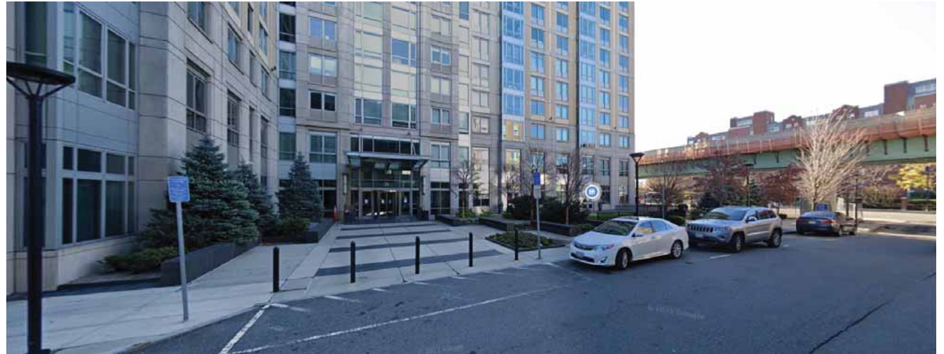
U.1 VIEW FROM LEIGHTON STREET OF WEST FACADE AND ELEVATED GREEN LINE
