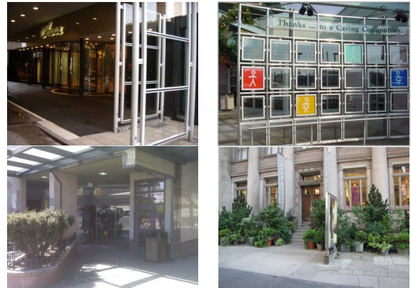
Image 10 – Wind Baffles for Building Entrances
