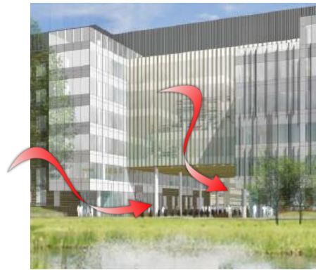
Image 8 – SW Winds Downwashing into the Passageway
