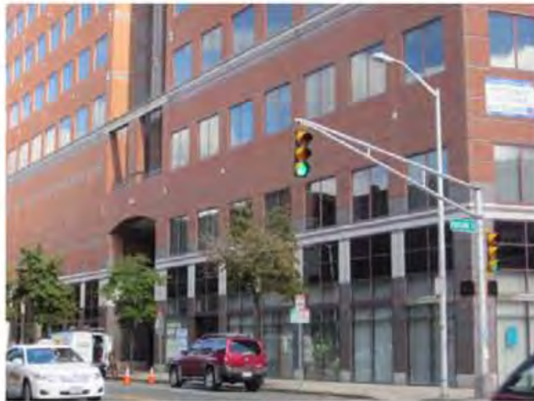
VIEW #191 BROADWAY AT PORTLAND ST
