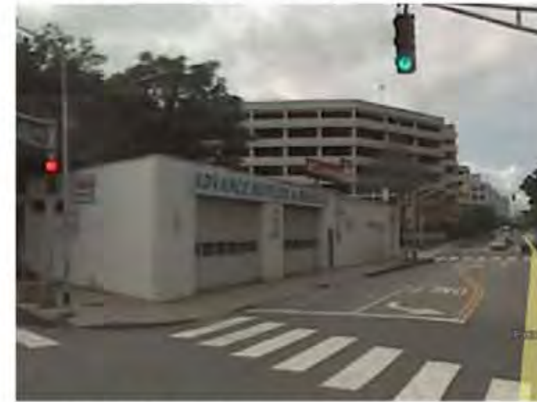
VIEW OF PORTLAND ST AT HAMPSHIRE ST
