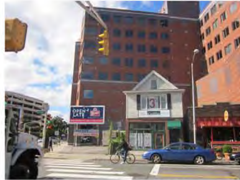
VIEW OF SITE, LOOKING SOUTH
