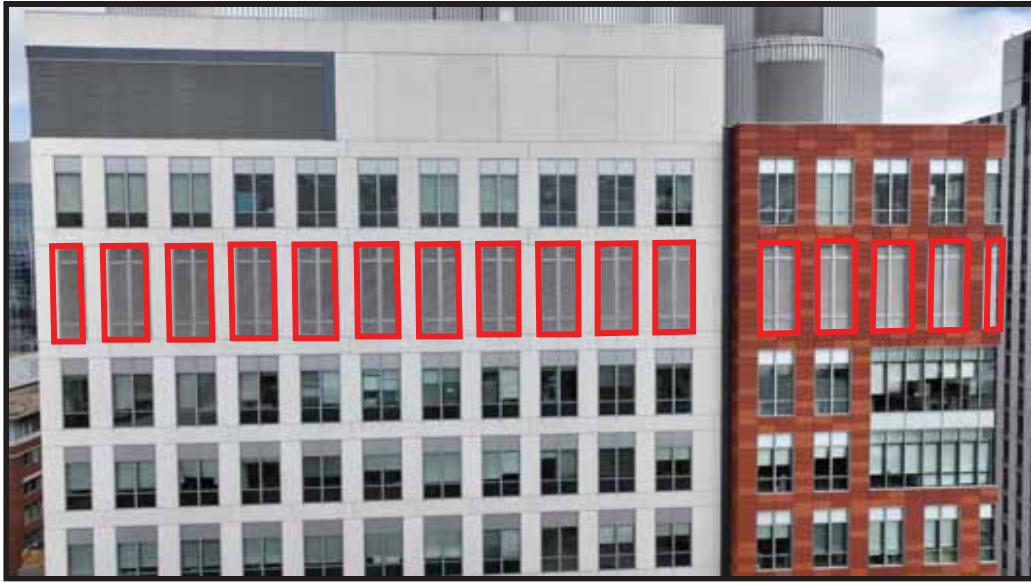
EXHIBIT D-1: OVERALL VIEW OF EXISTING FACADE. LEVEL M1 ANNOTATED RED
