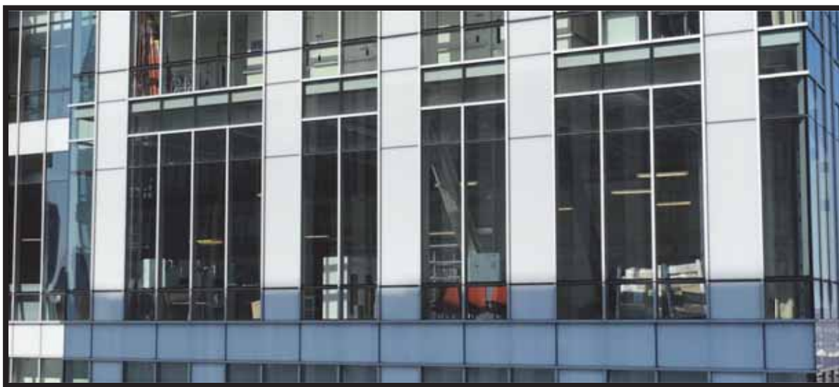
EXHIBIT C-2: ZOOMED IN VIEW OF CURTAINWALL CONDITION
