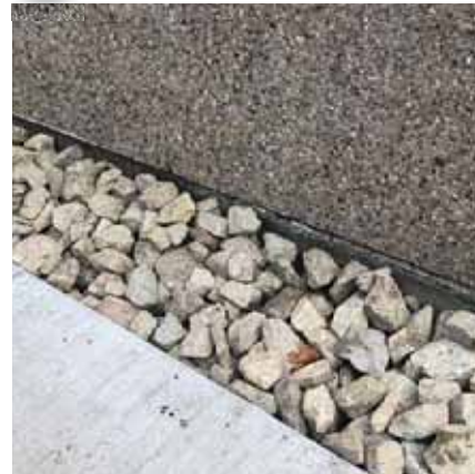
8 AGGREGATE DRIP STRIP
