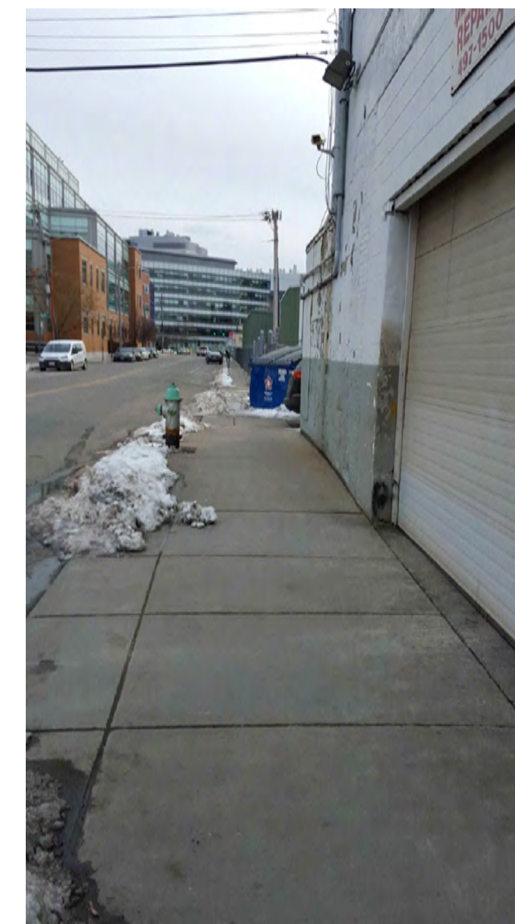
IMAGE 1-7. BUILDING FRONTAGE ALONG FULKERSON STREET
