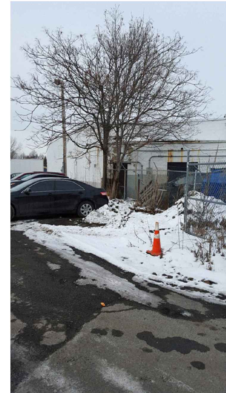
IMAGE 1-4. SOUTH END OF BUILDING AND ABUTTING PROPERTY
