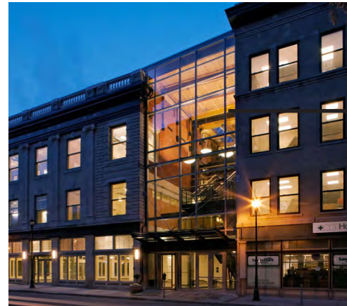
Existing masonry wall is featured through the glazing
