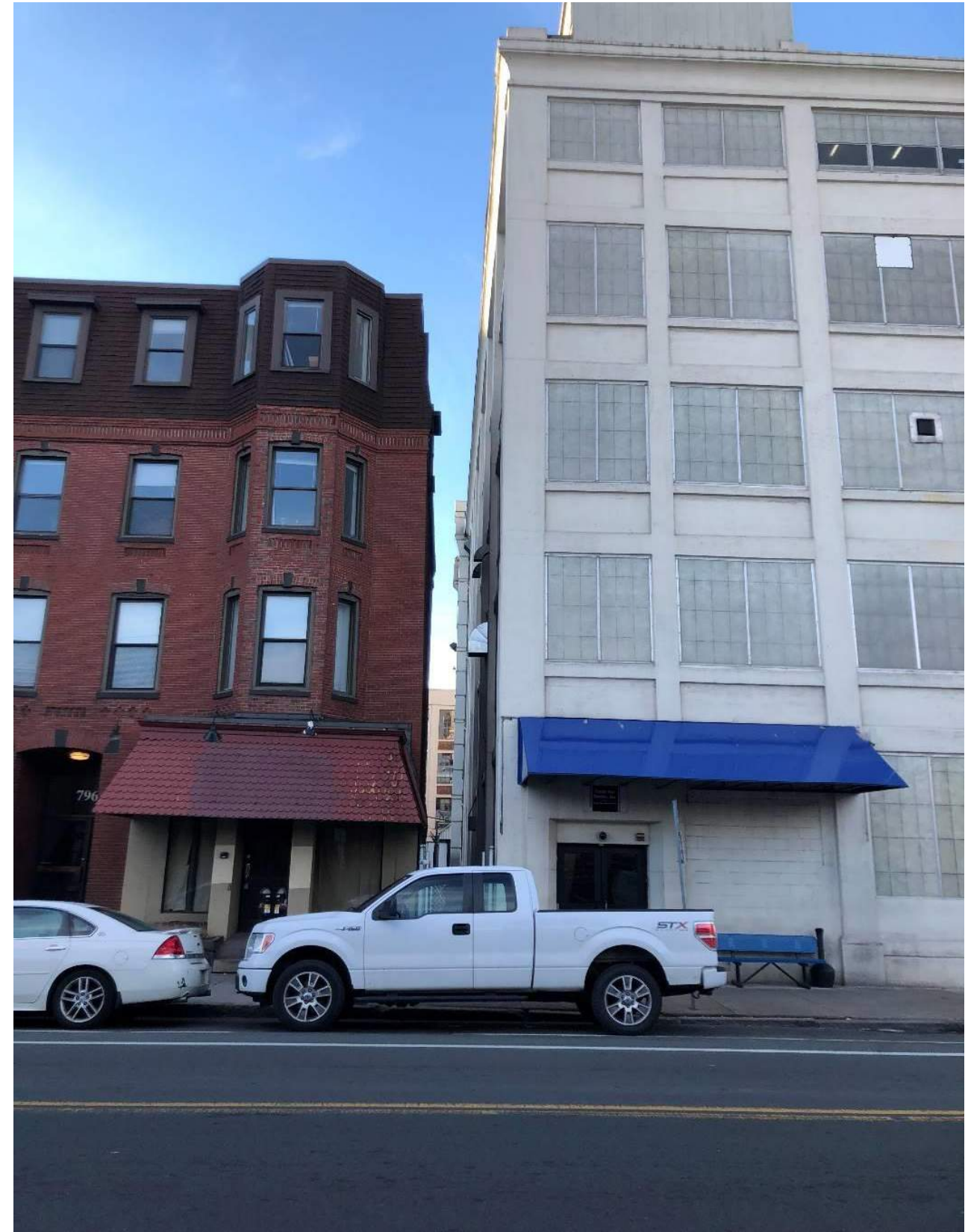
EXISTING CONDITIONS PHOTOGRAPHS: NEIGHBORING STRUCTURES
