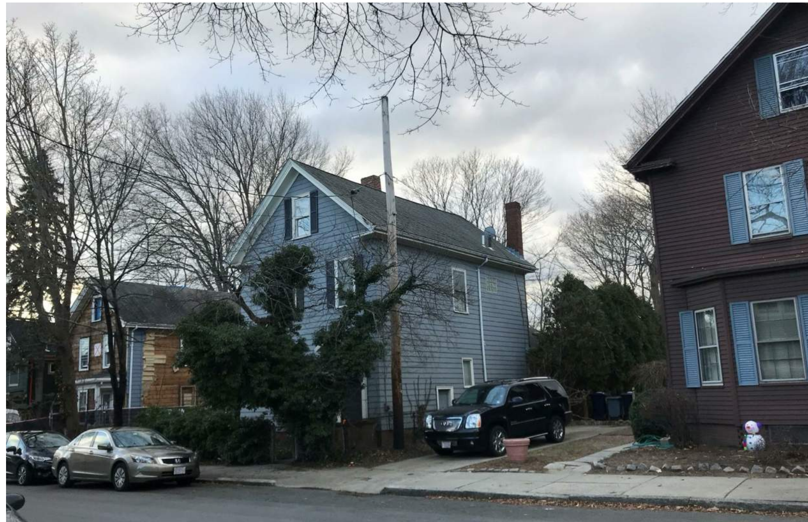
118 HOLWORTHY- RIGHT SIDE OF EXISTING HOUSE
