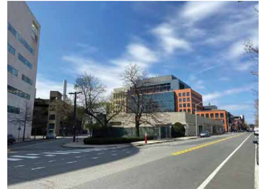
North side of Main St, looking Southwest towards Albany St
