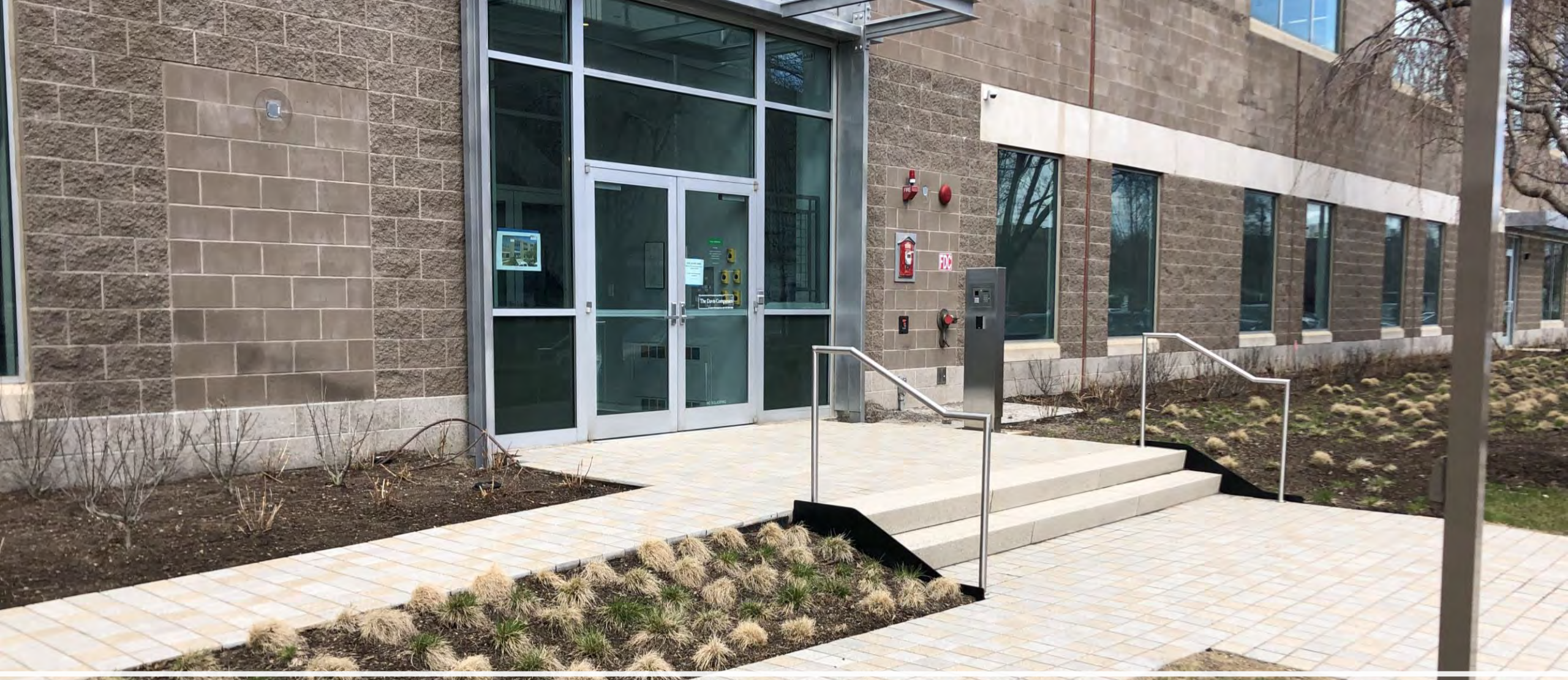
10 Wilson Road Main Entry (Café entry in distance on right)
