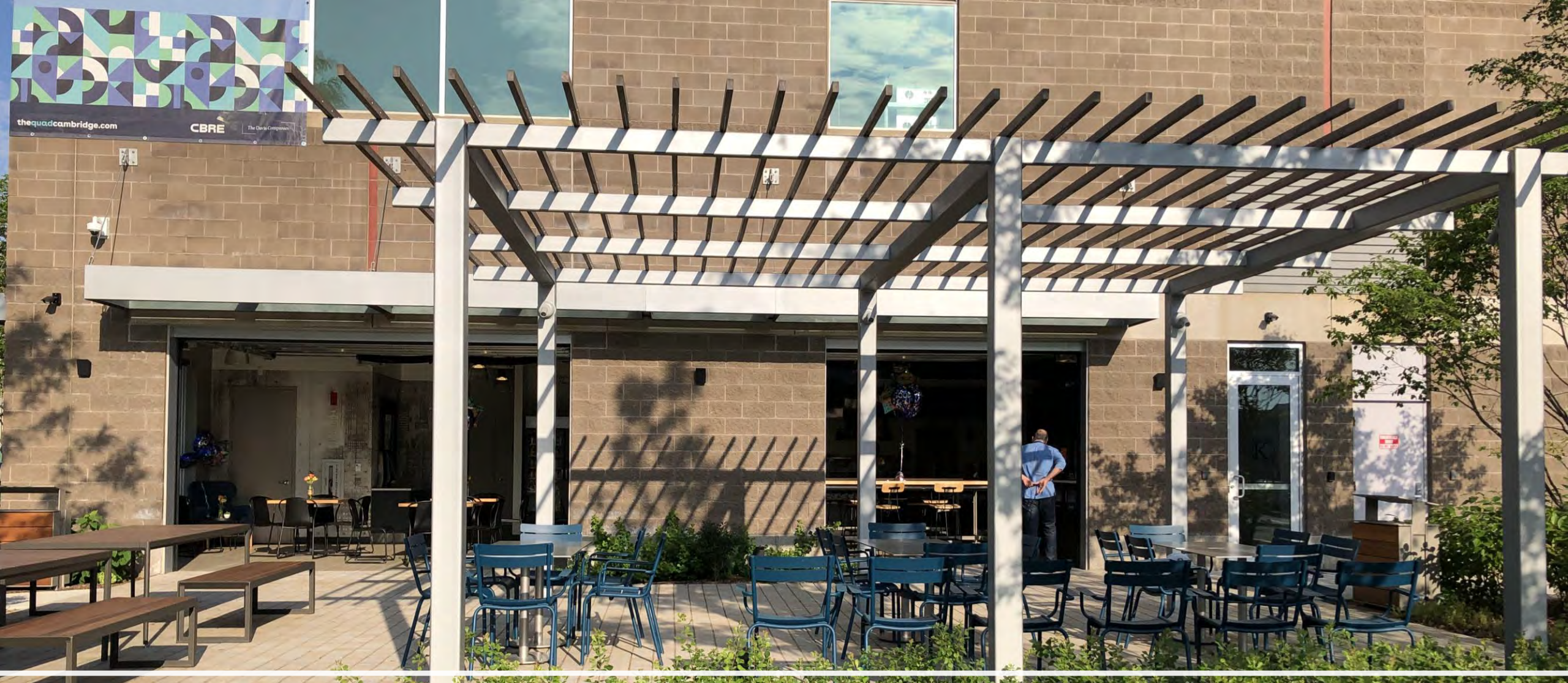
From Pocket Park, facing east façade 10 Wilson Rd
