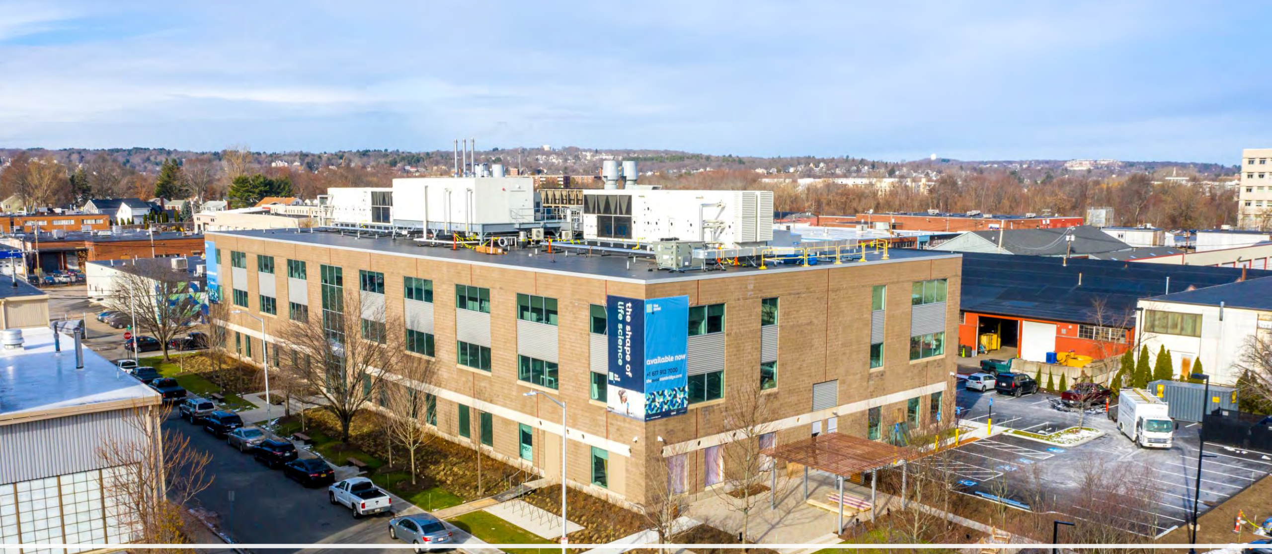
10 Wilson Road (from East)
