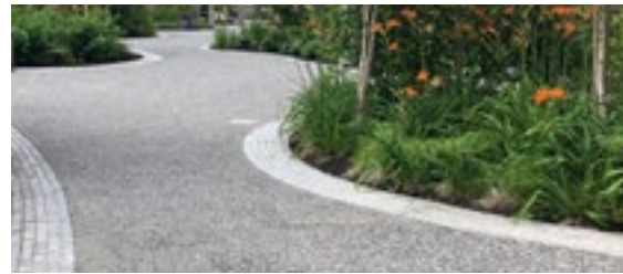
② Exposed Aggregate Concrete Pavement
