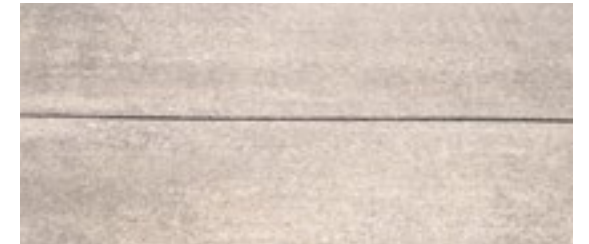
⑥ Concrete Pavement
