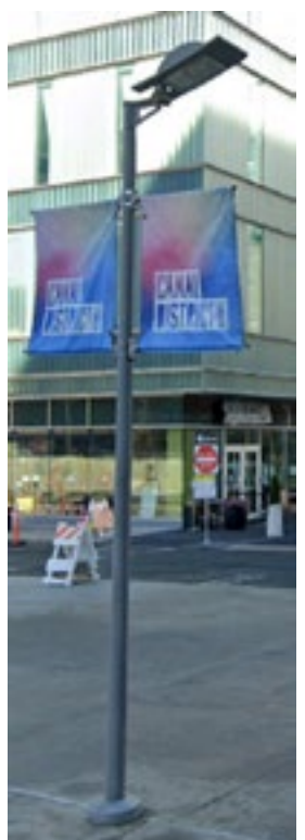
3 LP-K: Kendall Street Light Pole
