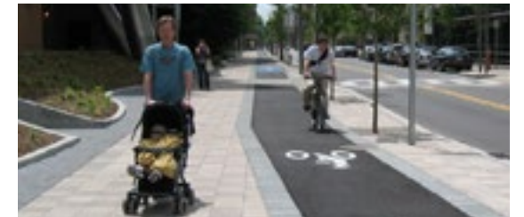
⑤ Bituminous Concrete Pavement (Raised Cycle Track)
