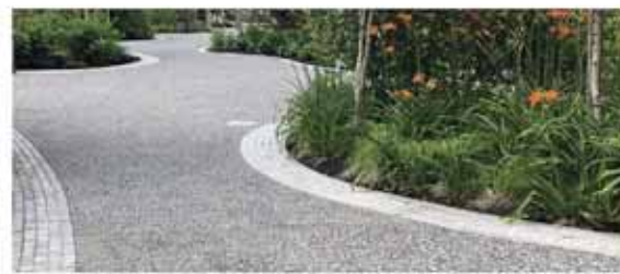
② Exposed Aggregate Concrete Pavement
