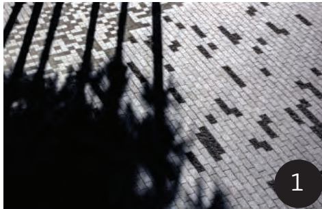
1 PRECAST PERMEABLE PAVERS
