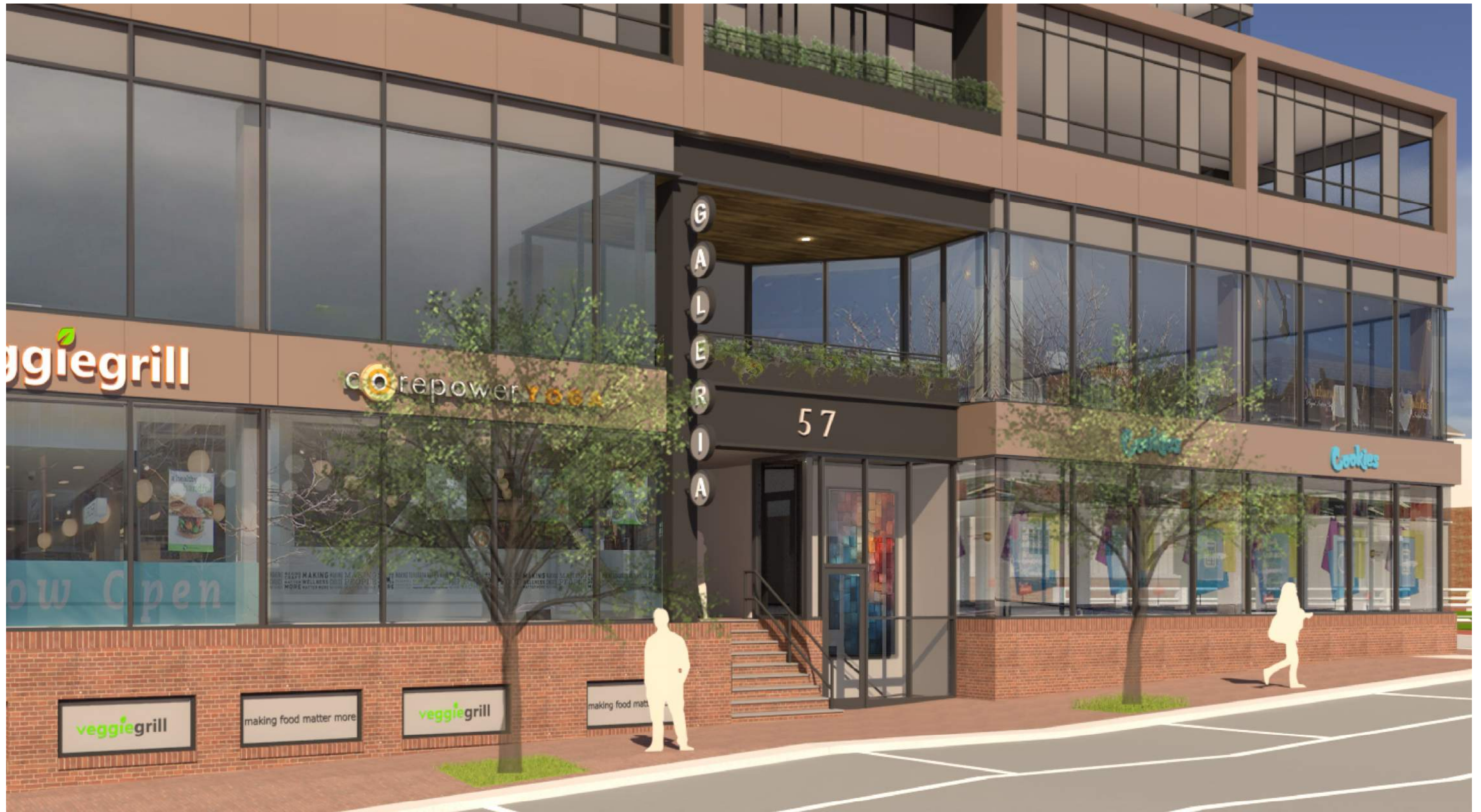
EXTERIOR BALCONY AT SECOND FLOOR DARK BRONZE COLORED ACM SPANDRELS AND COLUMN ENCLOSURE MOSAIC PANEL ON REAR WALL OF NEW ENTRY TO BASEMENT TENANT
