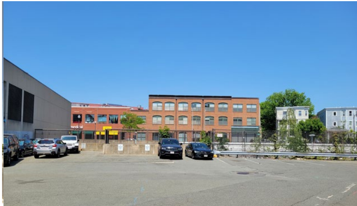
VIEW OF EXISTING BUILDING LOOKING NORTHEAST ACROSS COMMUTER RAIL
