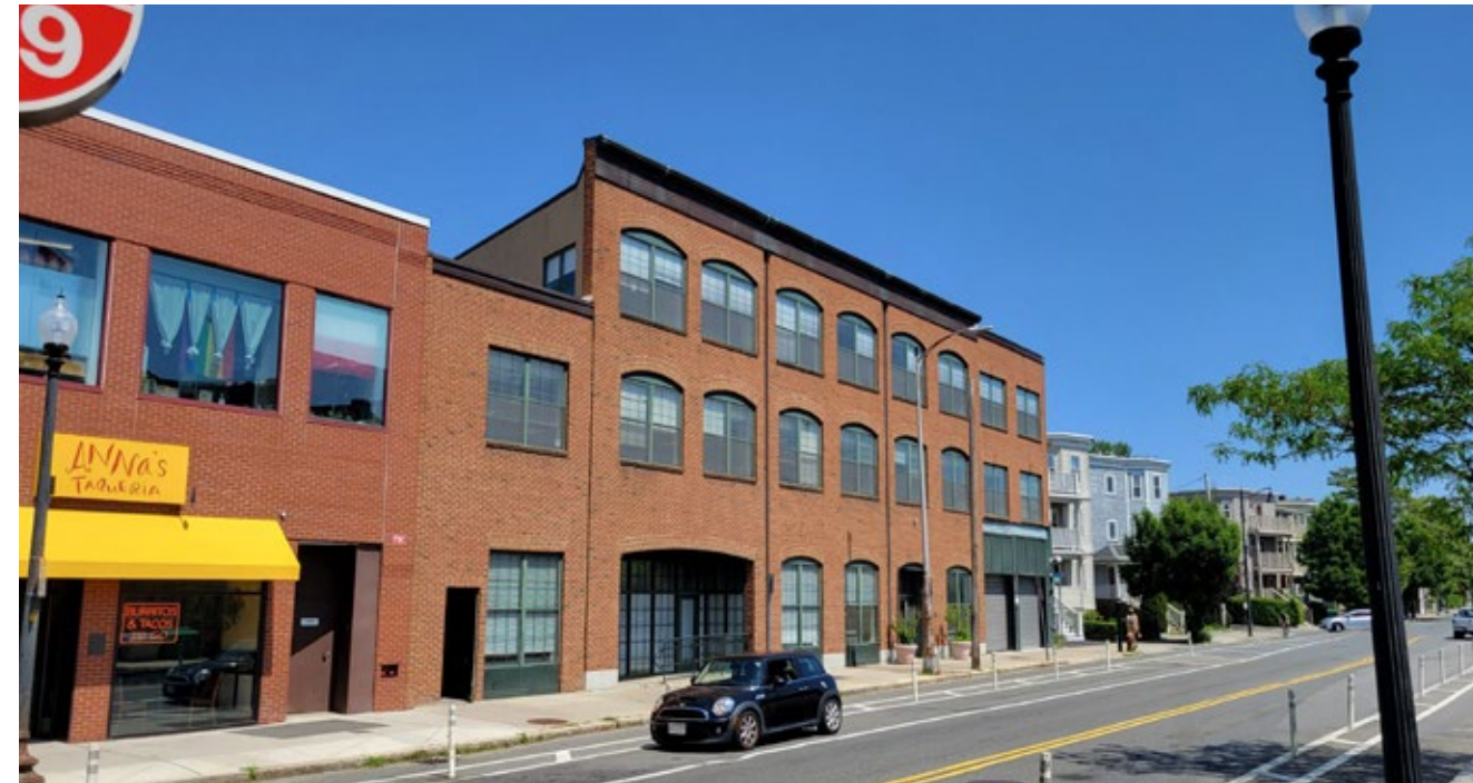
VIEW OF EXISTING BUILDING LOOKING SOUTH
