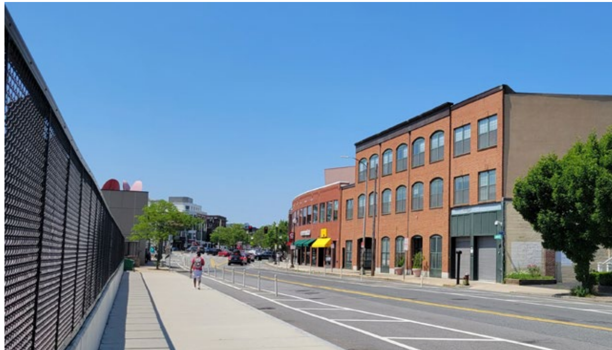
VIEW OF EXISTING BUILDING LOOKING NORTH
