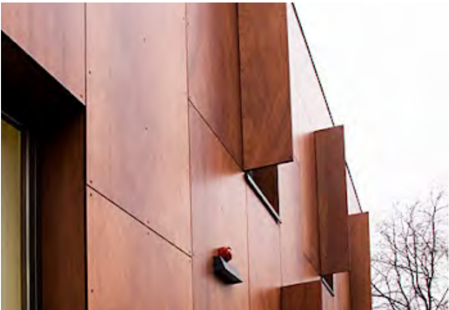
real wood veneer phenolic panel open joint install w/ exposed fasteners to match panel color
