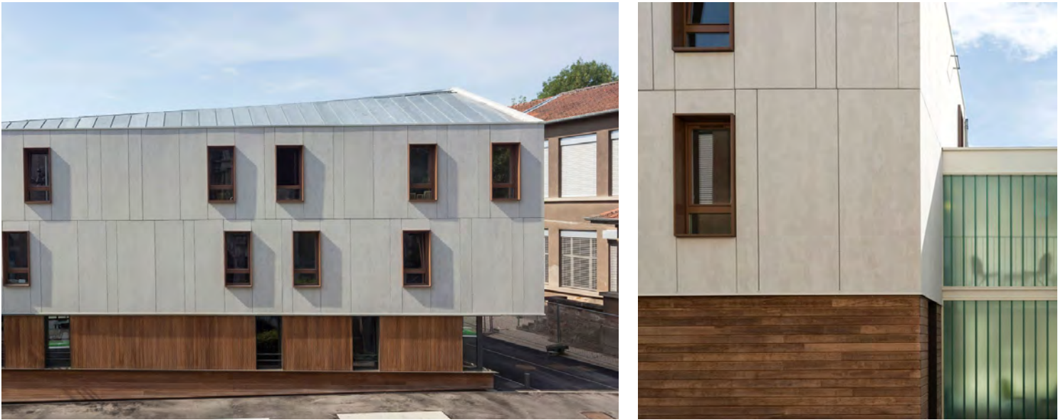
The cementitious panel has a natural quality to it that has both textural graining and sheen, with subtle tonal variations within each color. The large format panel application keeps a proportionate scale to the facades.
