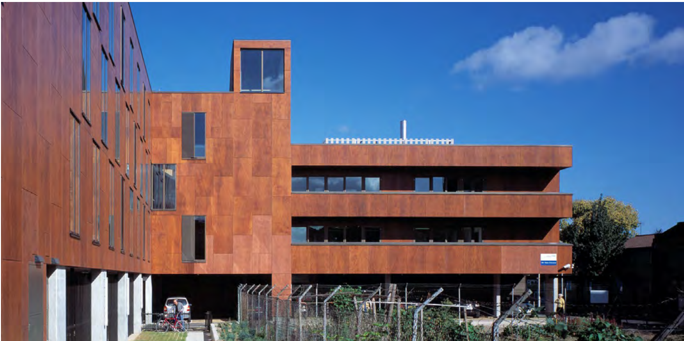
The phenolic panels contain real wood veneer, which gives inherent variation and richness to the facades. The application at New St varies from thinner slat panels to larger format panels at the New St plaza, where the full character of the graining will shine through.
