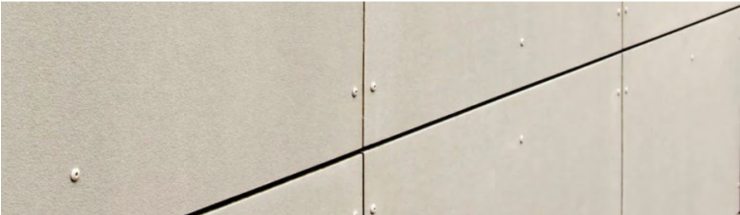
open joint install w/ exposed fasteners to match panel colors
