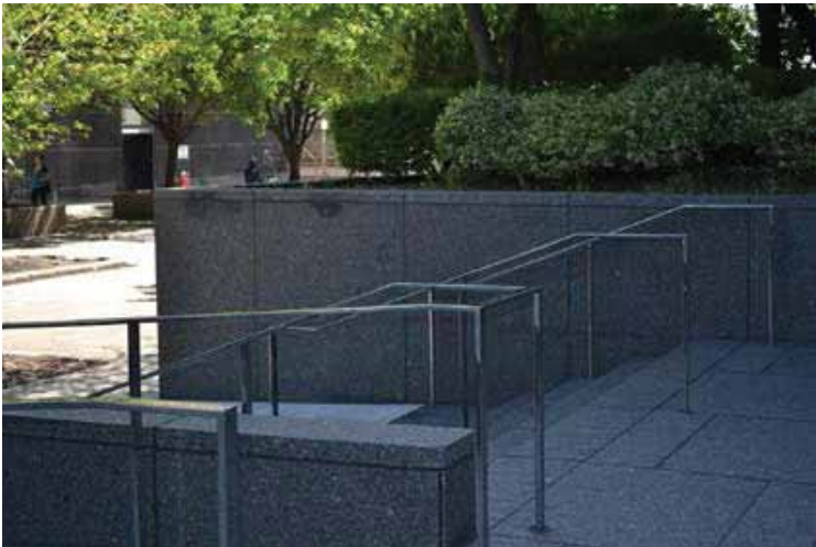
Granite Steps with Stainless Steel Handrail
