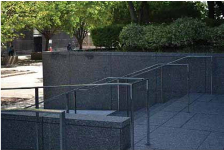
Granite Steps with Stainless Steel Handrail
