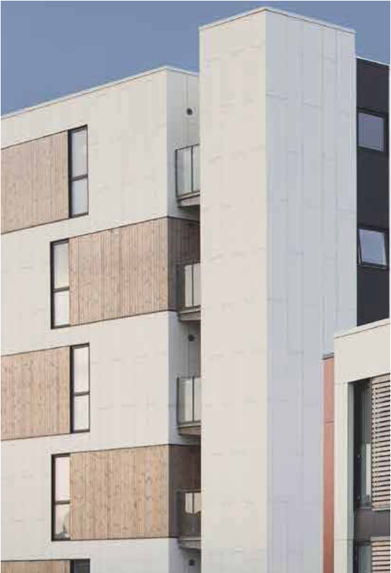
vertical wood look phenolic plank accents open joint install w/ exposed fasteners to match panel color
