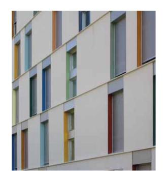
Fiber cement return in windows in varying colors, expresses the depth of the Passive House facade assembly
