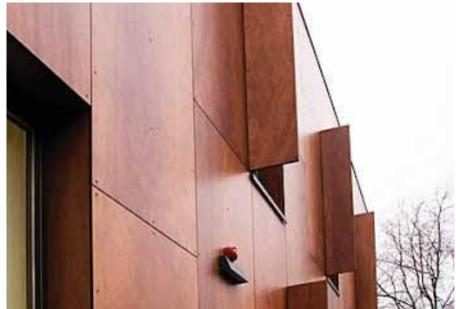
real wood veneer phenolic panel open joint install w/ exposed fasteners to match panel color
