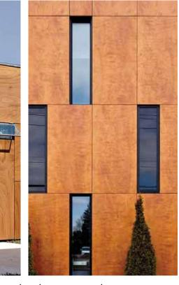
The phenolic panels contain real wood veneer, which gives inherent variation and richness to the facades. The application at New St varies from thinner slat panels to larger format panels at the New St plaza, where the full character of the graining will shine through.
