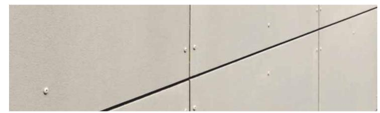
open joint install w/ exposed fasteners to match panel colors
