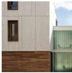
The cementitious panel has a natural quality to it that has both textural graining and sheen, with subtle tonal variations within each color. The large format panel application keeps a proportionate scale to the facades.
