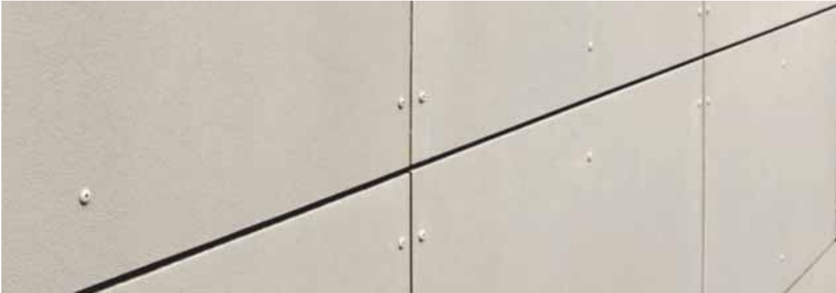
earth tone cementitious panels - two sets of gradient colorways open joint install w/ exposed fasteners to match panel colors
