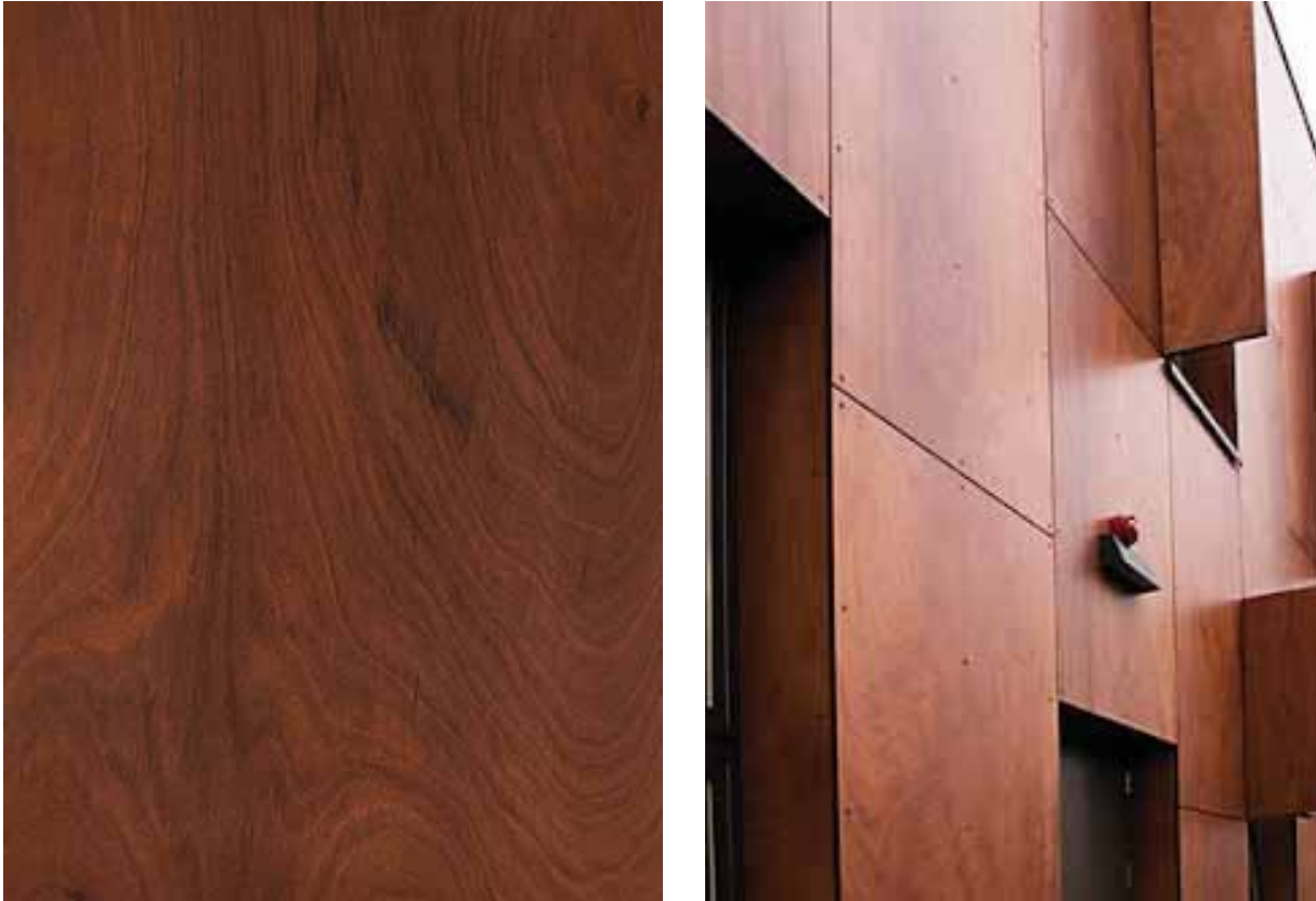
wood panel accents open joint install w/ exposed fasteners to match panel color
