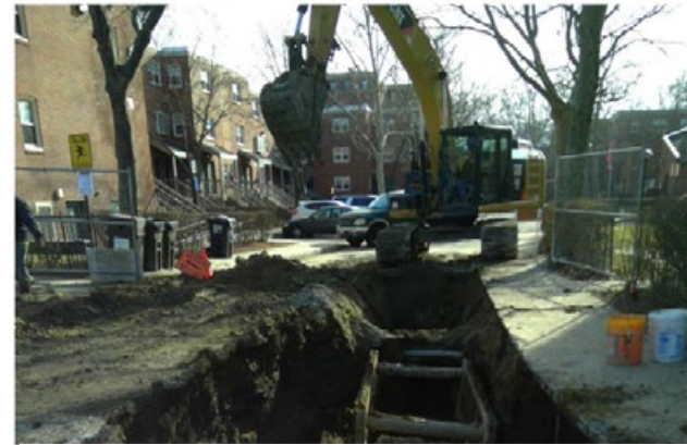
Figure 4: All existing buildings suffer from failing utilities such as deteriorating sewer pipes and water mains causing flooding onsite.
