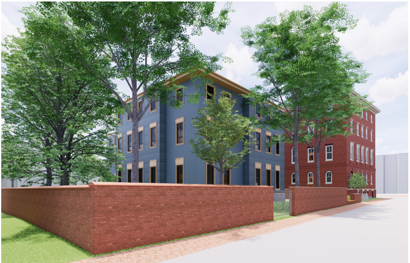
Figure 9: View of north facade from Worcester Street. Fiber cement shingles and fiber cement clapboards alternate at the recesses and projections. Ground-face CMU will be installed at the base of the building. Colors have not been chosen yet, but neutral warm tones will be used.
