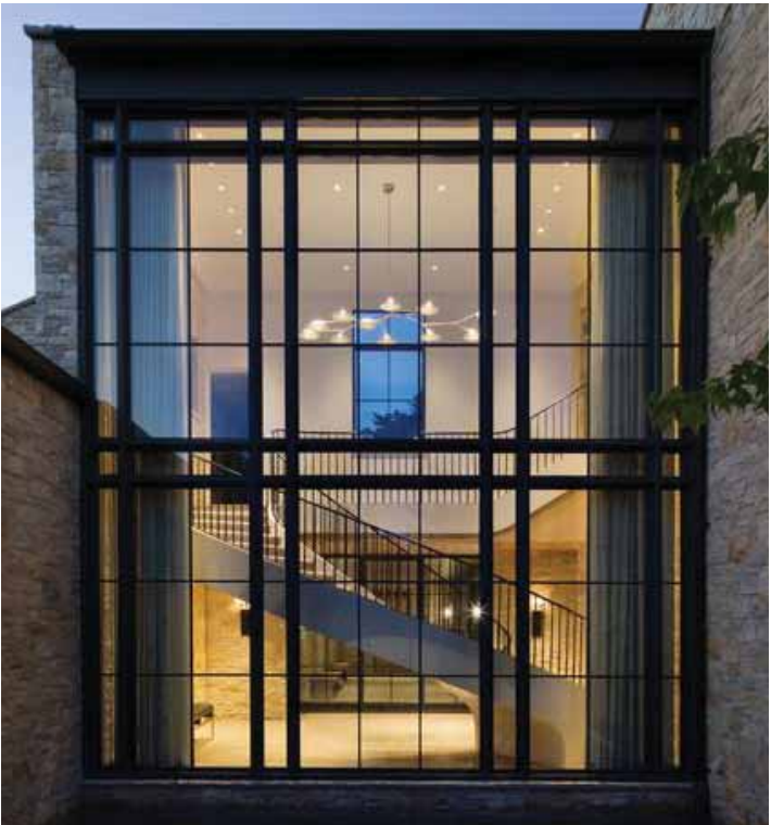
Curtainwall connector between existing building and addition
