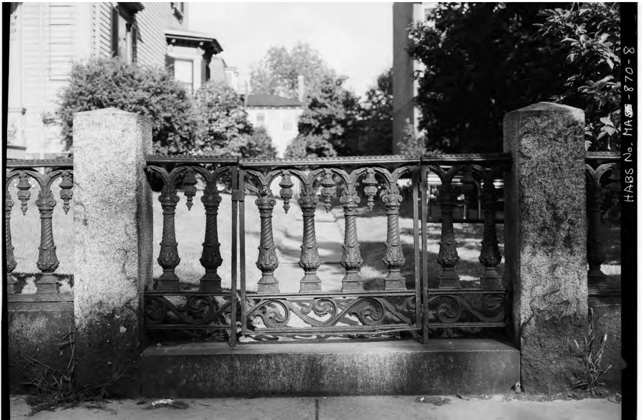
Cast iron fence and gate at Massachusetts Avenue. HABS photo, 1964.
