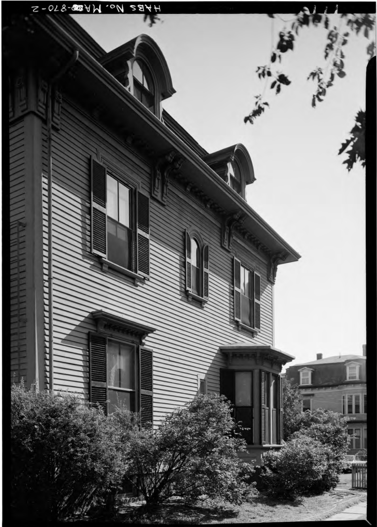
South elevation, from the southeast. HABS photo, 1964.
