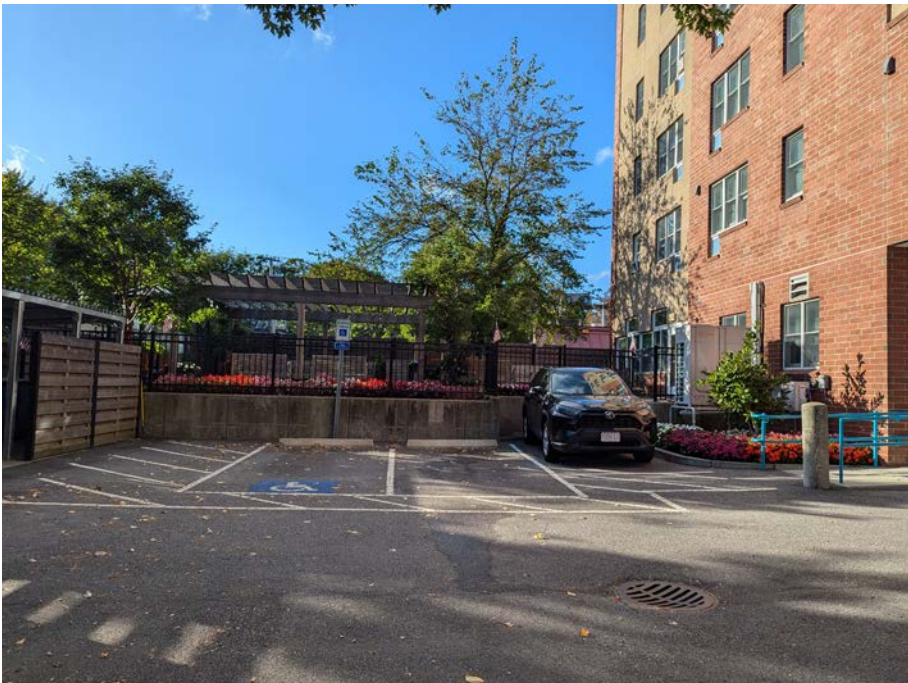
RUSSELL APARTMENT COMMUNITY GARDEN AND PARKING LOT
