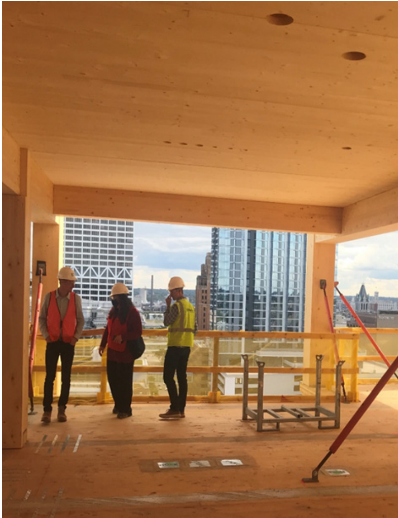
Mass Timber project under construction
