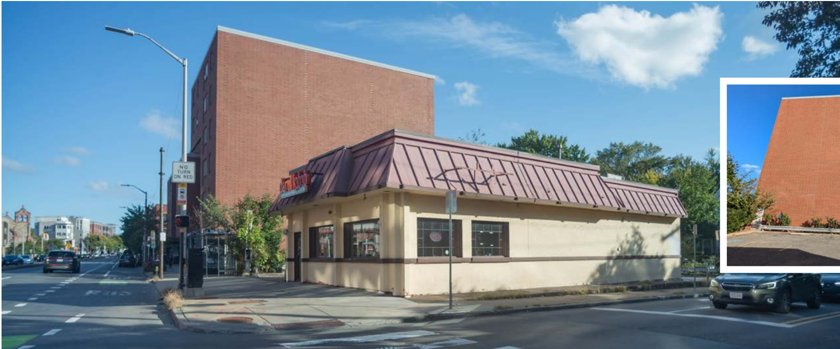
SIX-STORY BLANK BRICK WALL FACING NORTH CAMBRIDGE
