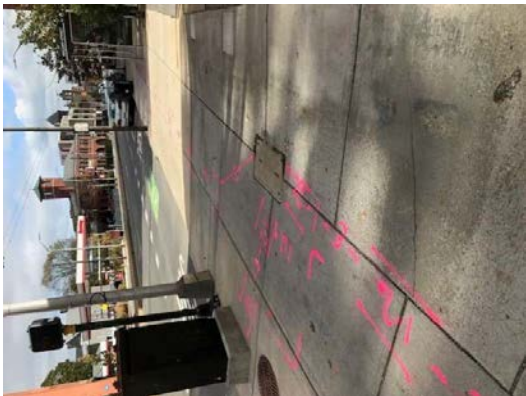
Possible signal control or site lighting located 1-2 feet from the surface, extending in both directions down Mass Ave.
