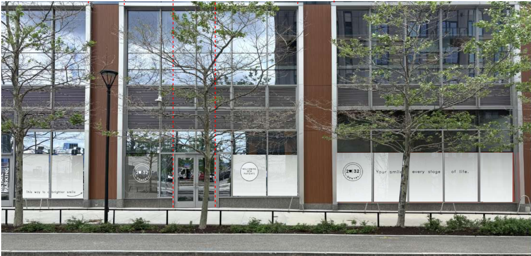
WINDOW FILM WILL BE APPLIED TO THE INTERIOR SURFACE OF THE GLASS AS REQUIRED FOR HIPAA COMPLIANCE AS REGULATED BY THE DEPARTMENT OF HEALTH AND HUMAN SERVICES (HHS) TO PROTECT THE IDENTITY AND PROTECTED HEALTH INFORMATION (PHI) OF PATIENTS.
