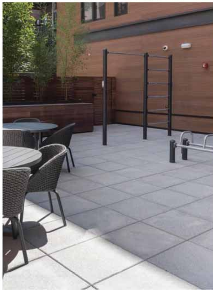
PRECAST PAVERS ON PEDESTALS
