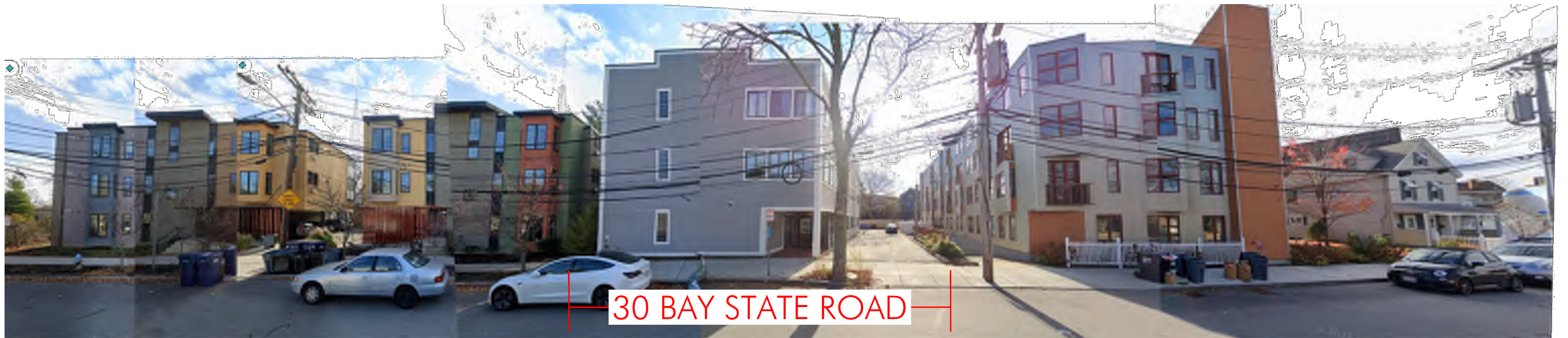
BAY STATE ROAD (SOUTH)
