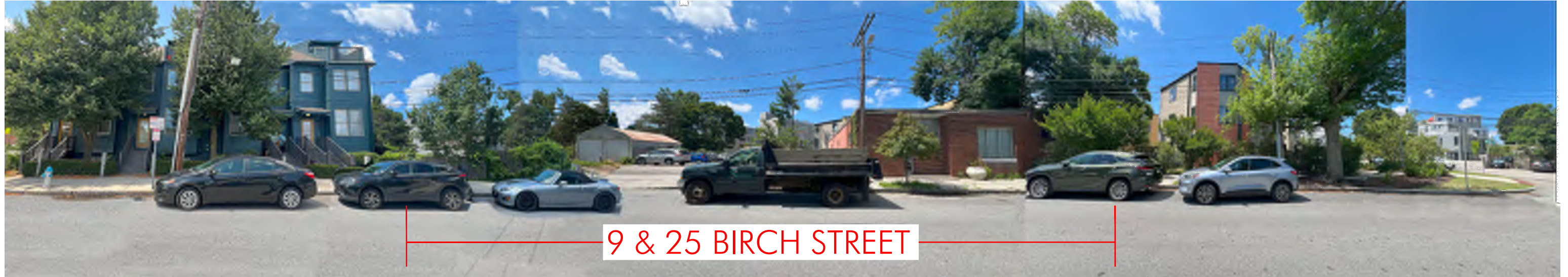
BIRCH STREET (NORTH WEST)
