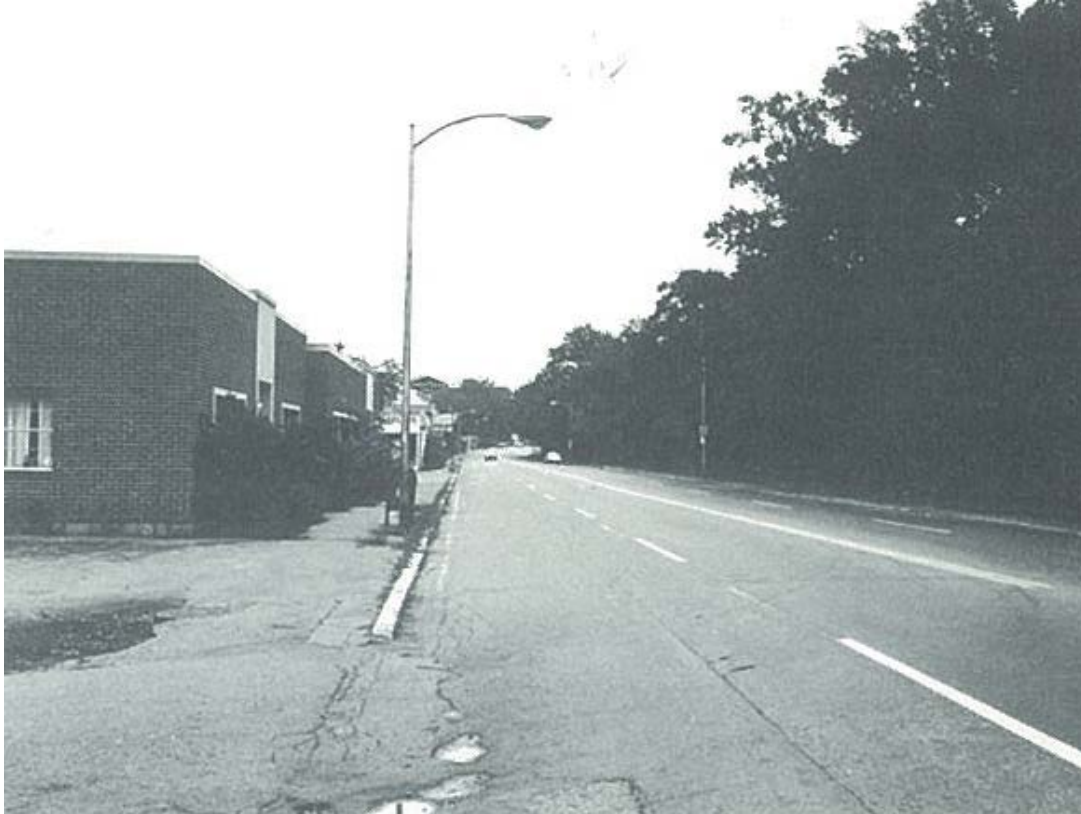
Roadway lack adequate sidewalks, tree planting, and other public amenities / 1979. (Source: Alewife Revitalization. Alewife Urban Design Study Phase II)
