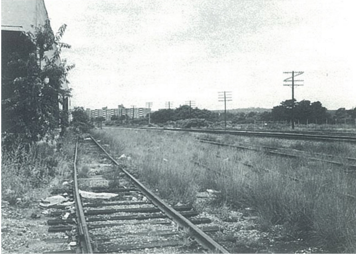
Underutilized Railroad Yards / 1979. (Source: Alewife Revitalization. Alewife Urban Design Study Phase II)
