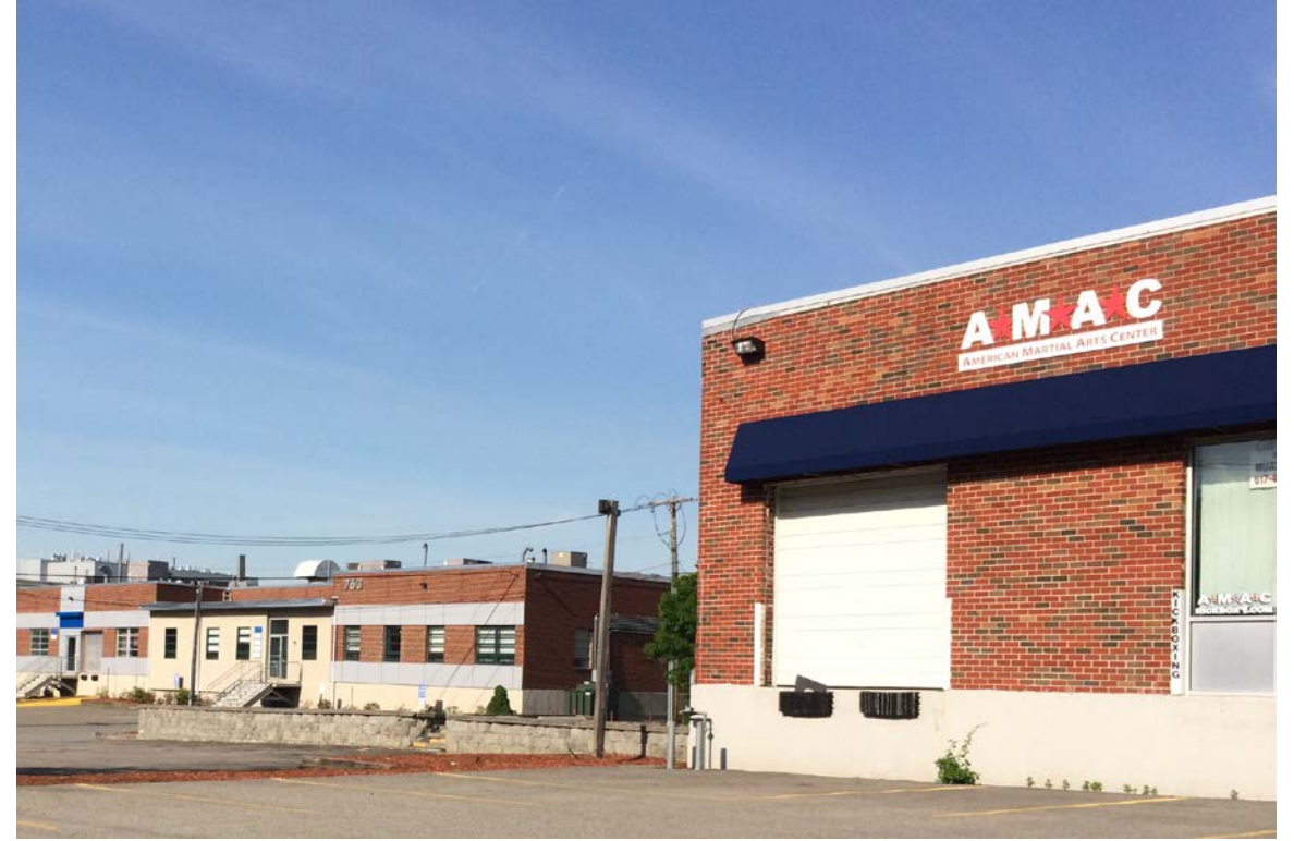
Industrial Buildings in Spinelli PI / 2016. (Source:)
