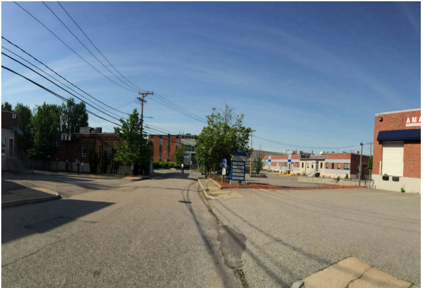
The Alewife Quadrangle has large amounts of impervious surface and little tree canopy, making it vulnerable to climate-related natural disasters.
